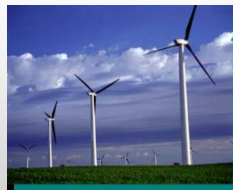
NSP 107 MW Lake Benton wind farm 4 cents/kWh (unsubsidized)
