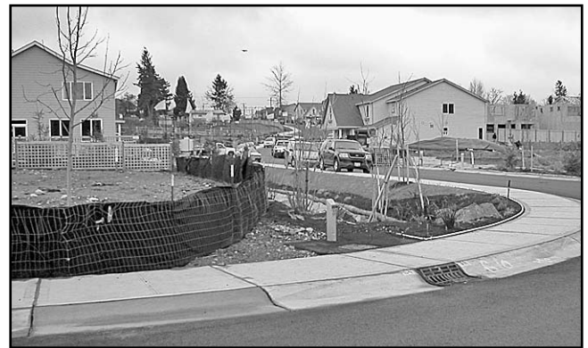
Erosion and sediment control measures in the new Shamrock Heights development east of Renton worked effectively during the 05-06 rainy season.
