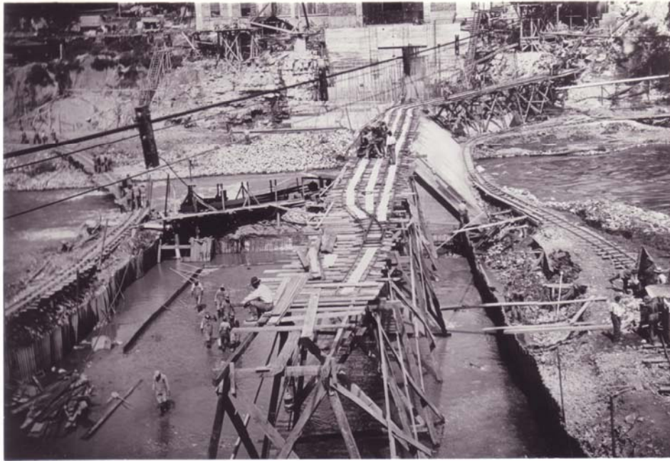
7/20/1911 – Concreting in mattress of east portion of dam.
