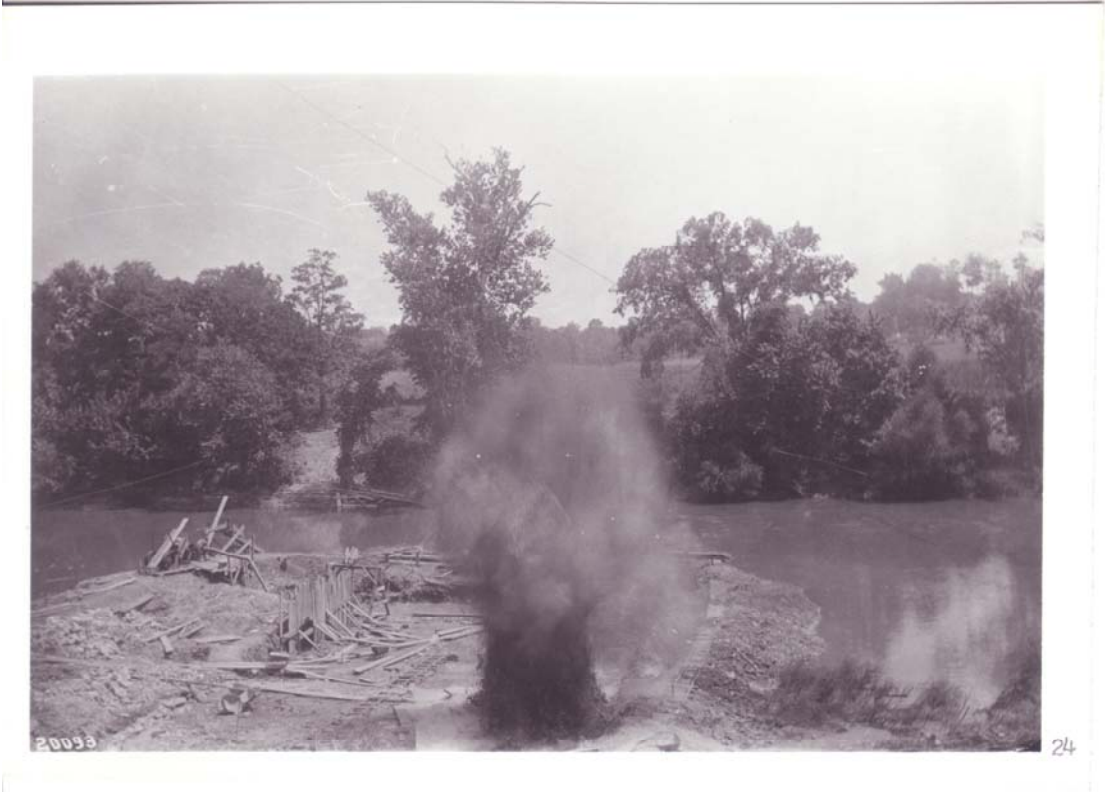
1910 – Williams Historic dam, construction photograph.
