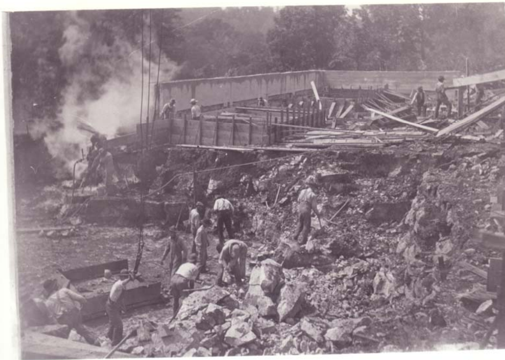
6/11/1910 -- Stone excavation in engine room. Drilling in progress.
