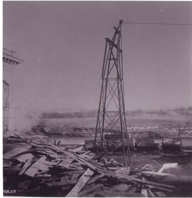
2/16/1911 – Testing strength of main transmission tower. View of tower after failure.
