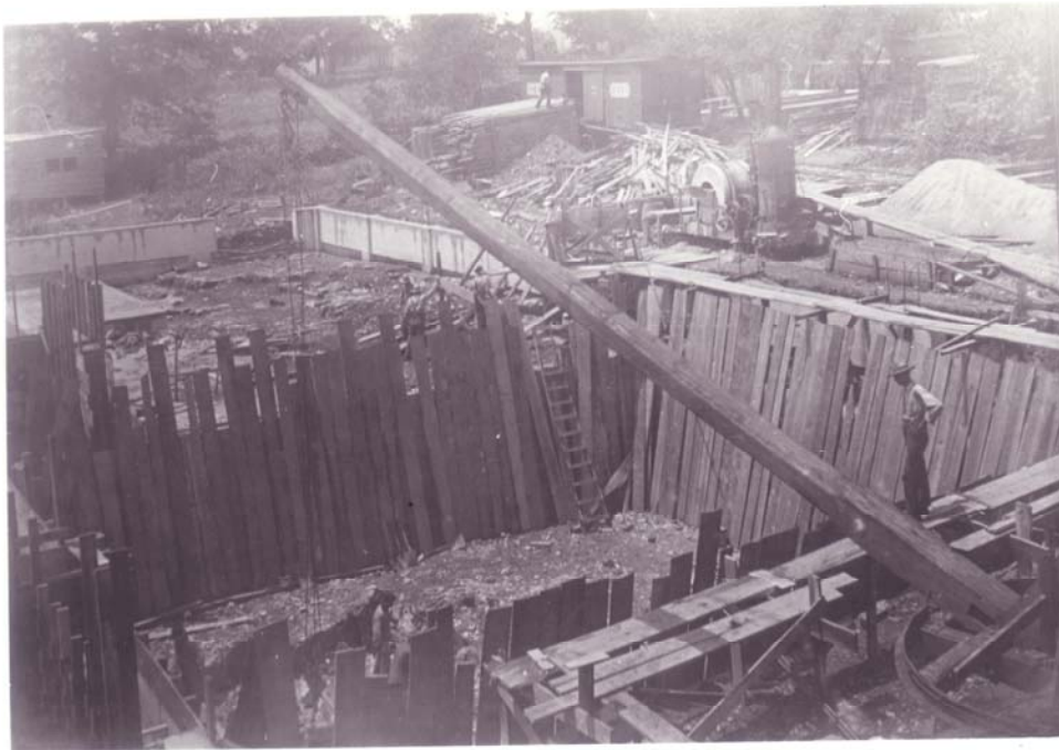
7/2/1910 – View from stone pile north end of power house.
