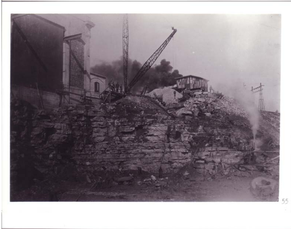
2/15/1911 – View of wheel pit excavations.
