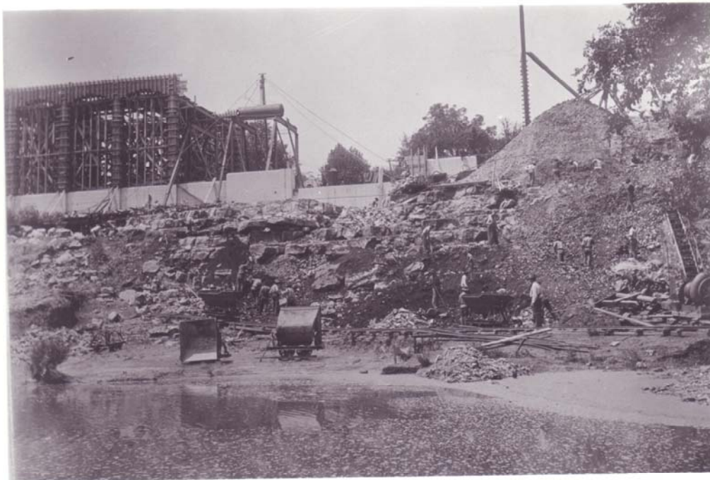
1910 – Williams Historic dam, construction photograph.
