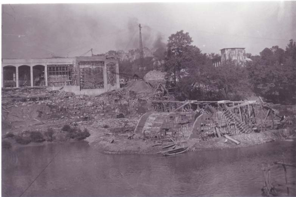
1910 – Williams Historic dam, construction photograph.
