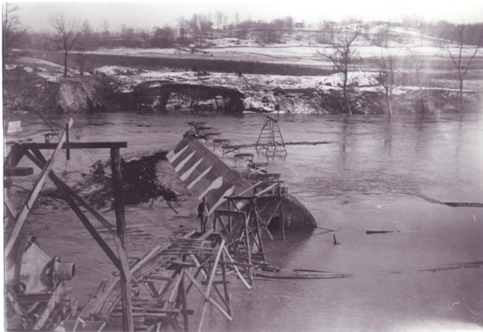
12/30/1910 – View of flood looking east from runway to mixer.
