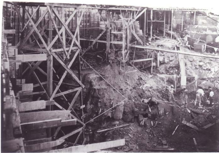
9/6/1911 – Mixing and distributing plant and machinery platform.
