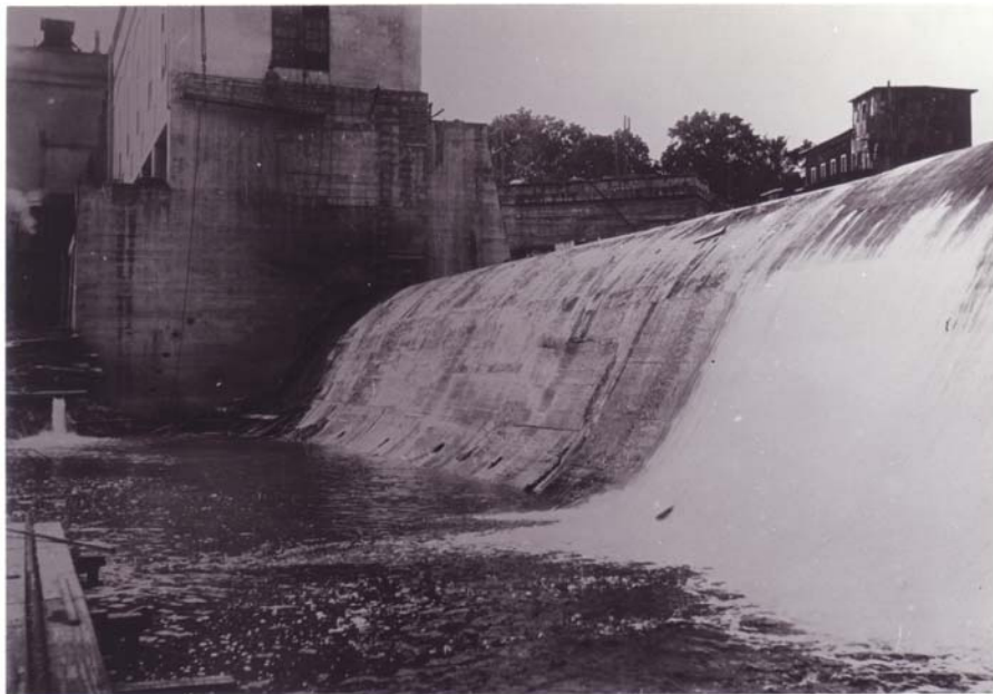
8/9/1912 – View showing repaired portion of dam on downstream side.
