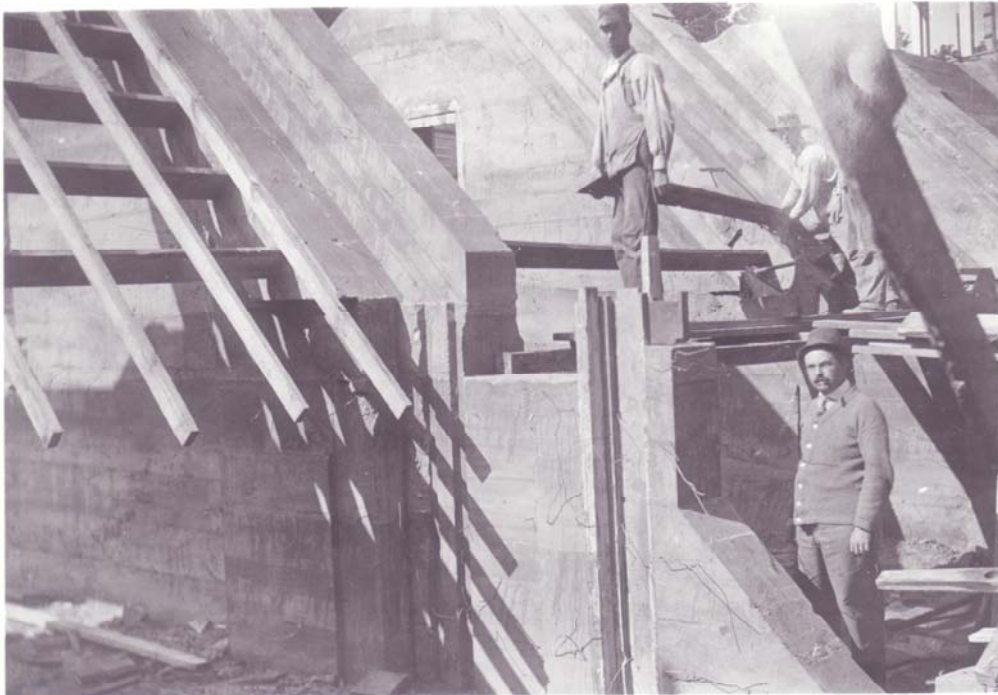
1910 – Williams Historic dam, construction photograph.
