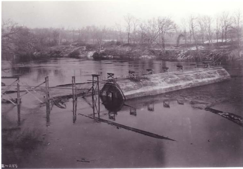
12/30/1910 – View looking northeast from southeast corner of boiler house.
