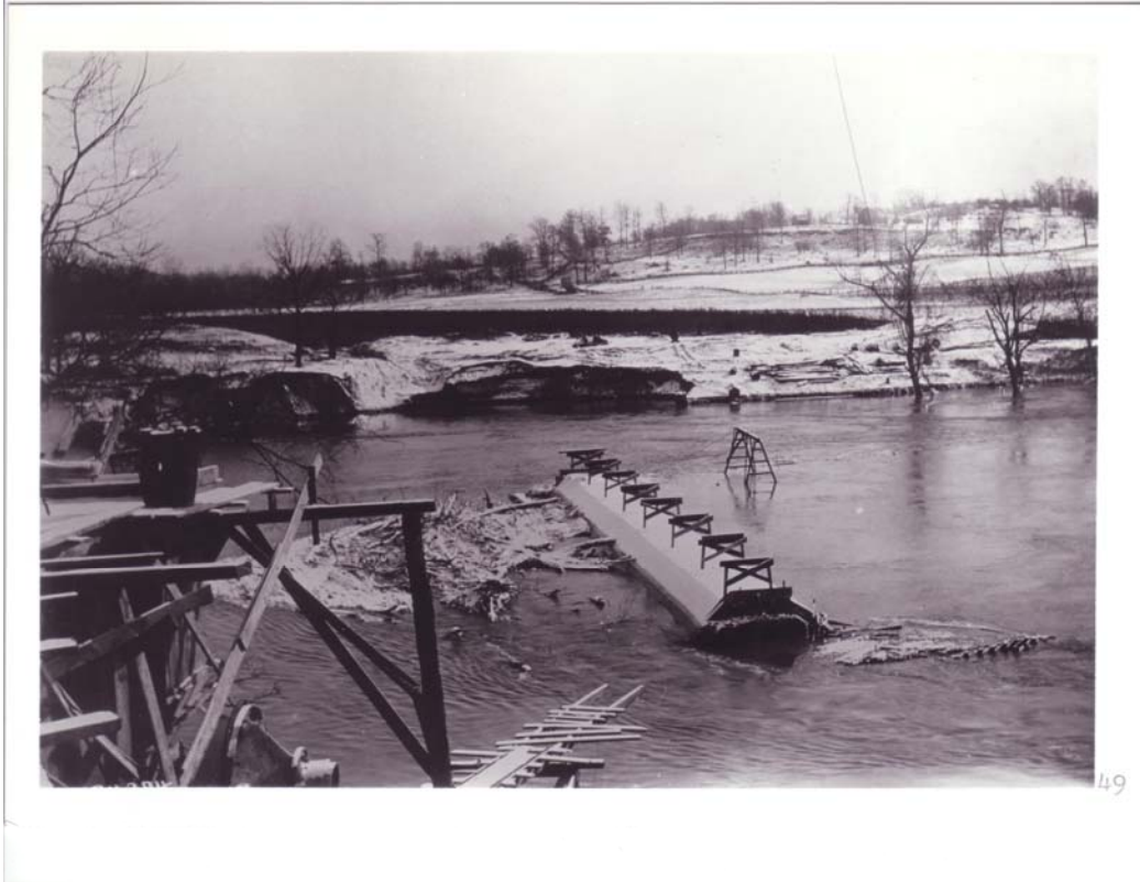
1/4/1911 – View of flood looking east from runway to mixer.
