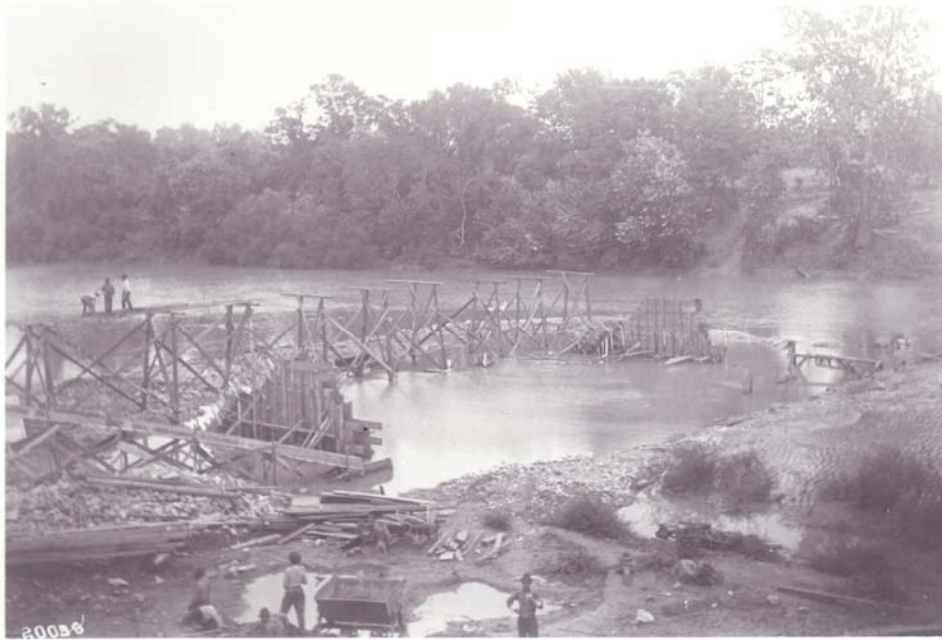
1910 – Williams Historic dam, construction photograph.
