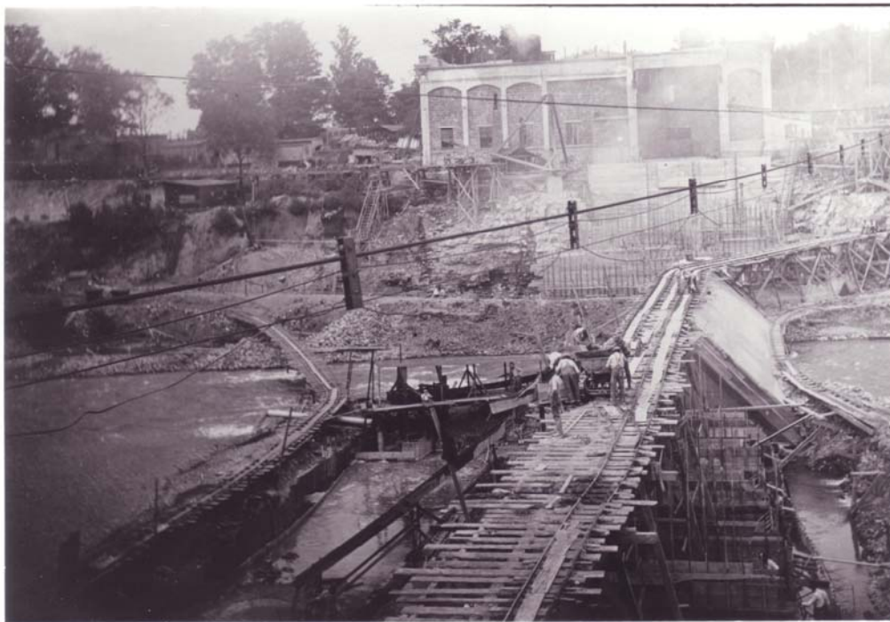
7/25/1911 – Concreting mattress of dam, showing buttress forms.
