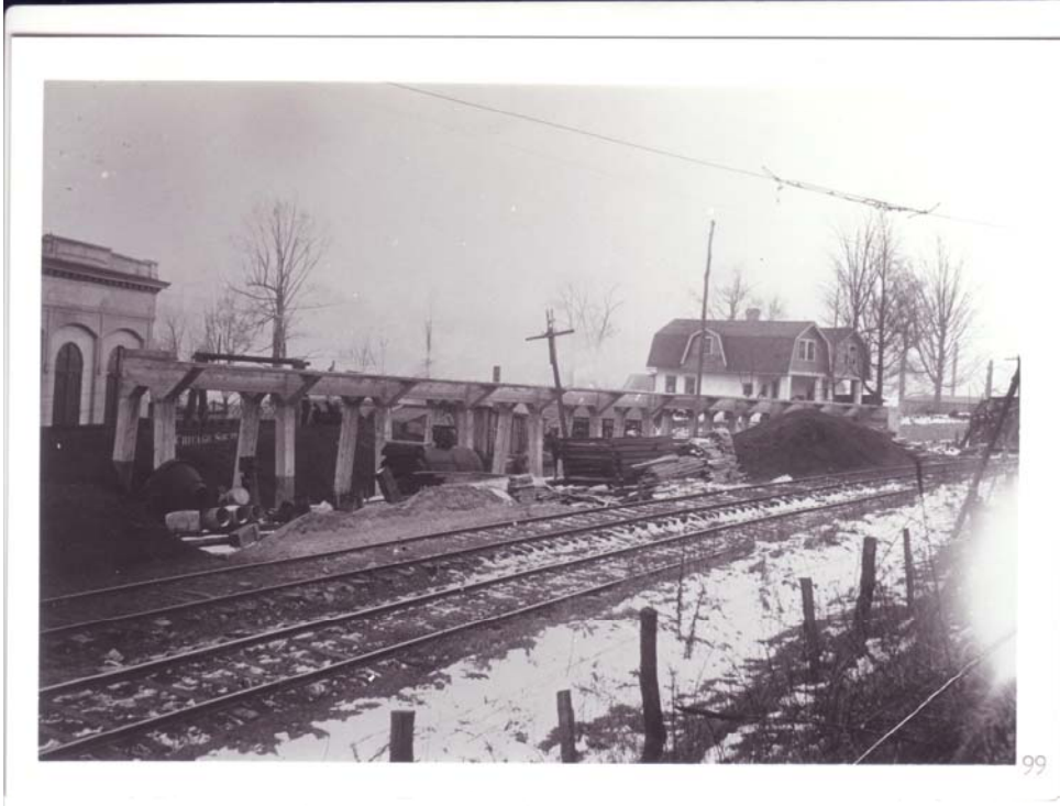
2/14/1912 – View of trestle from north end.
