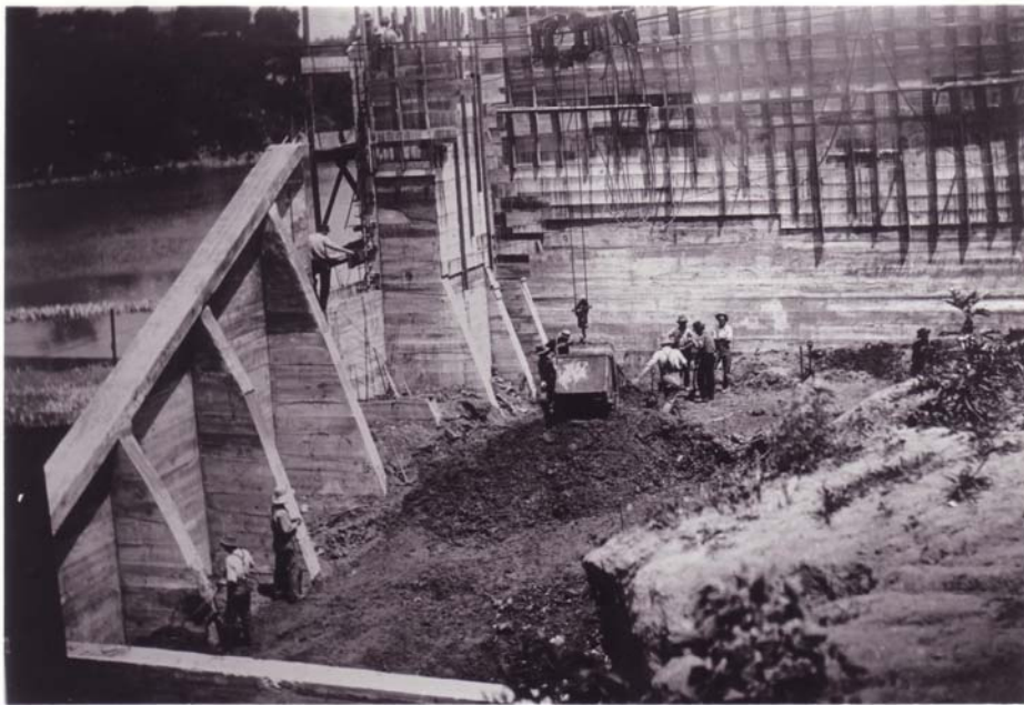
7/18/1911 – Abutment from rear showing back fill.
