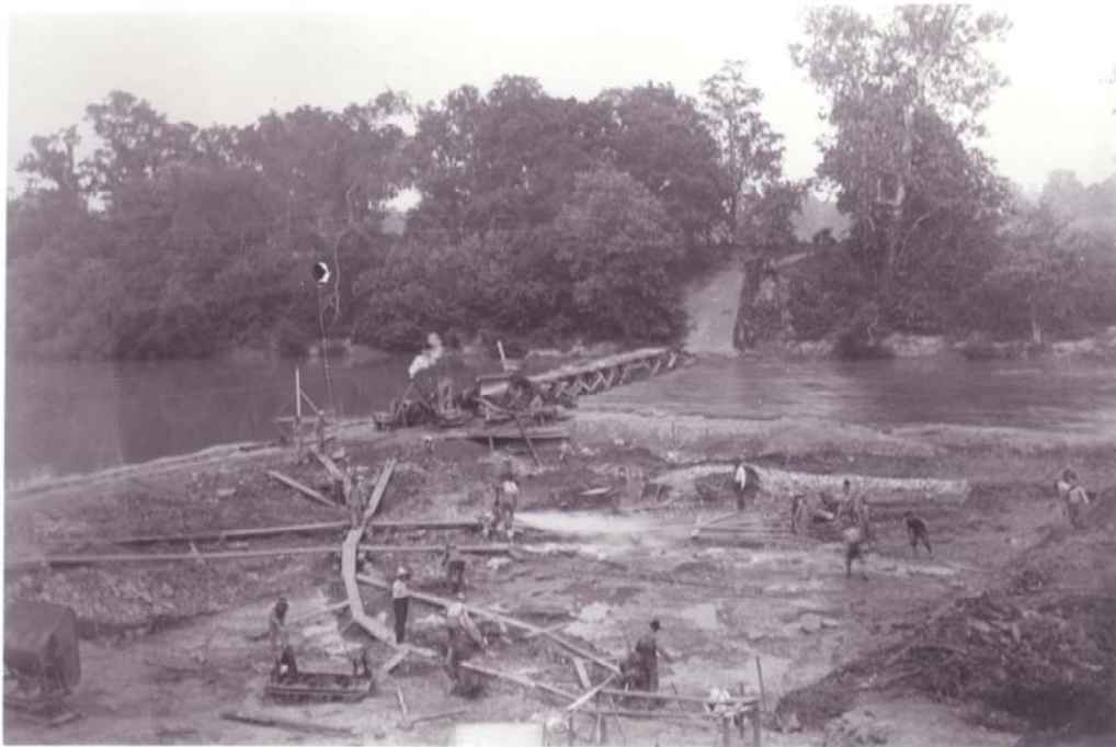
6/3/1910 – View of coffer dam from wheel pits.
