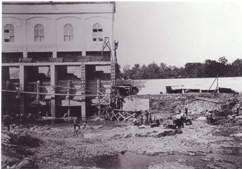
6/6/1912 – View of tail race excavation hole pumped out.
