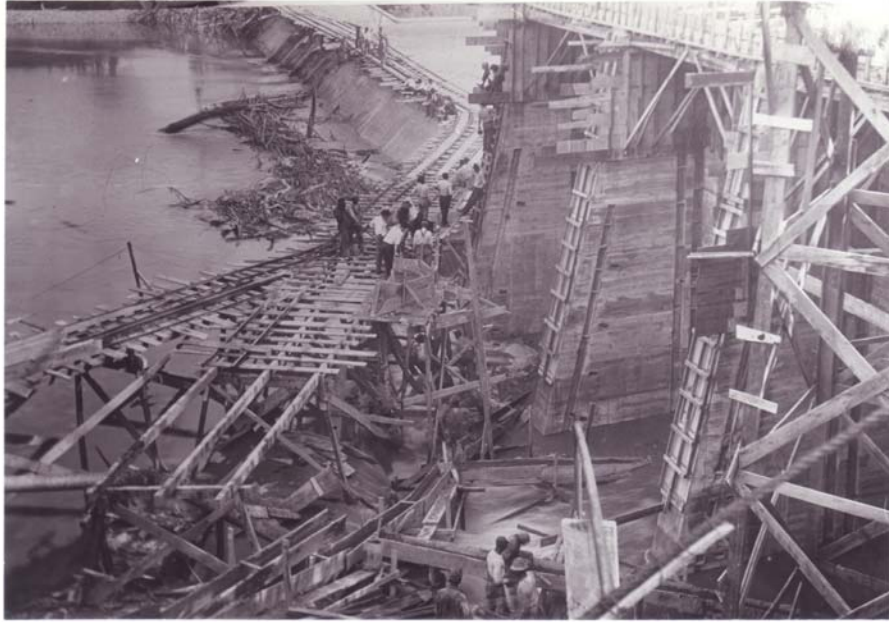
9/17/1911 – River over concrete coffer dam. Removing drift from cableway.
