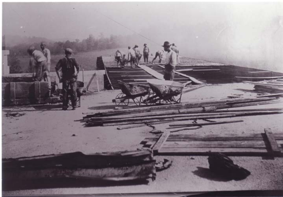
9/29/1911 – Concreting roof slab. Water wheel building.
