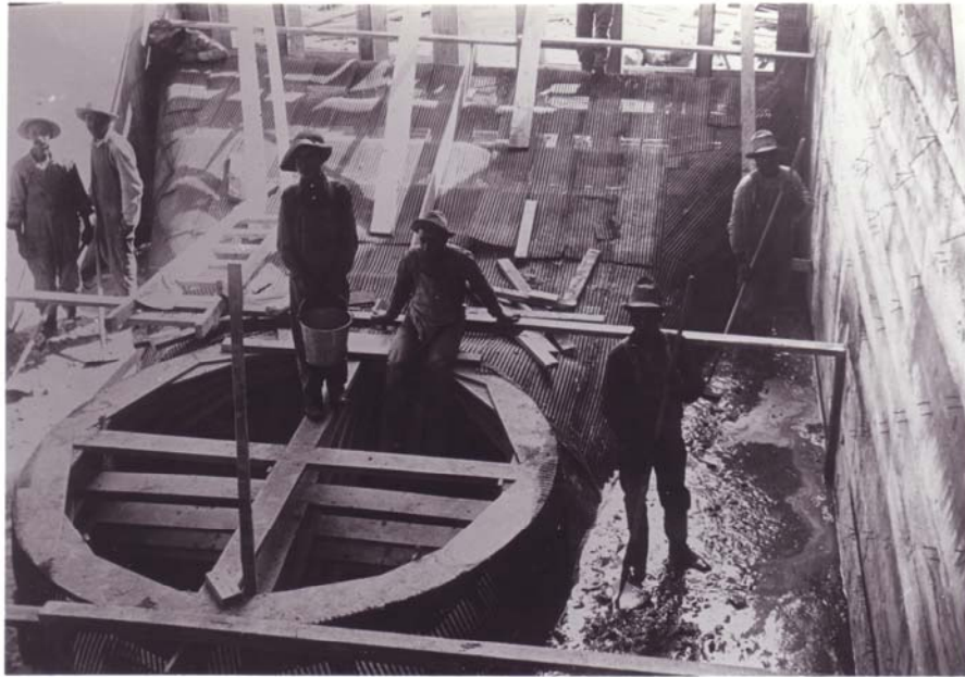
8/31/1911 – Concreting lower draft tube #3.
