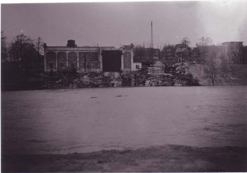
4/6/1911 – View of flood and buildings from opposite bank. Water elevation 476.
