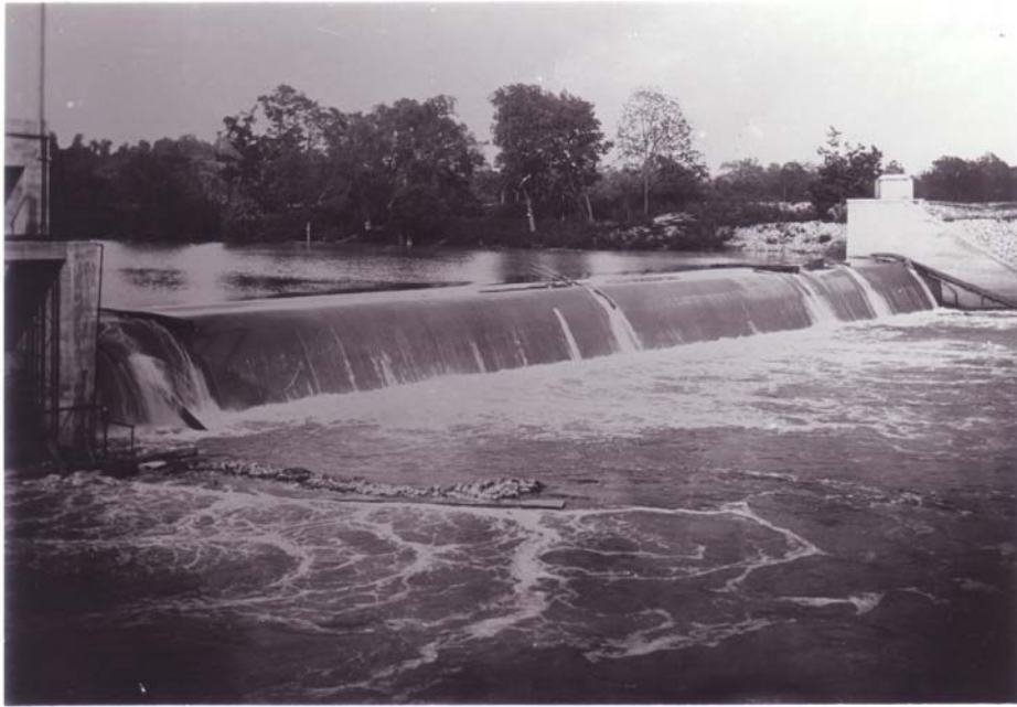
8/12/1912 – Showing spillway and tail race. Elevation tail water 461.9.
