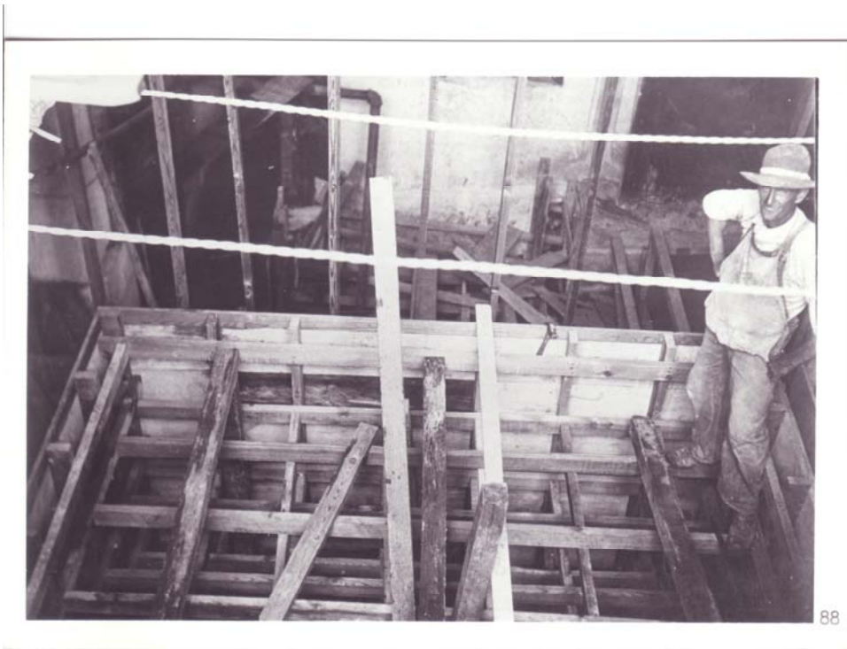
9/6/1911 – 1750 KW turbine foundation.
