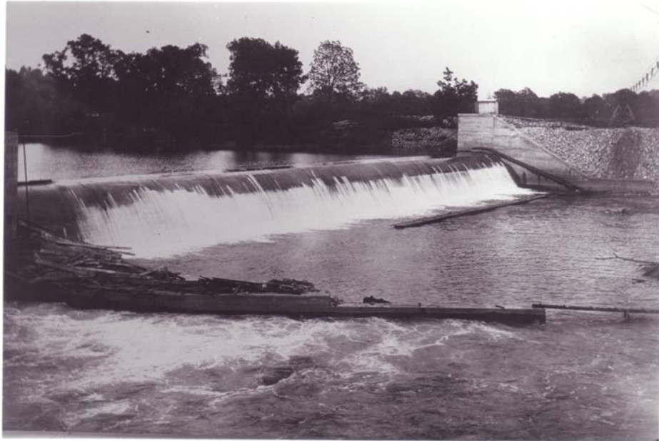
8/7/1912 – Water passing repaired portion of dam. Tail race elevation 459.
