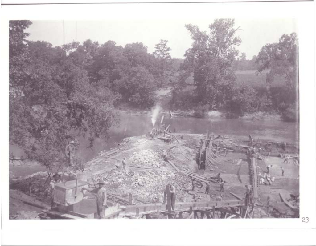
1910 – Williams Historic dam, construction photograph.
