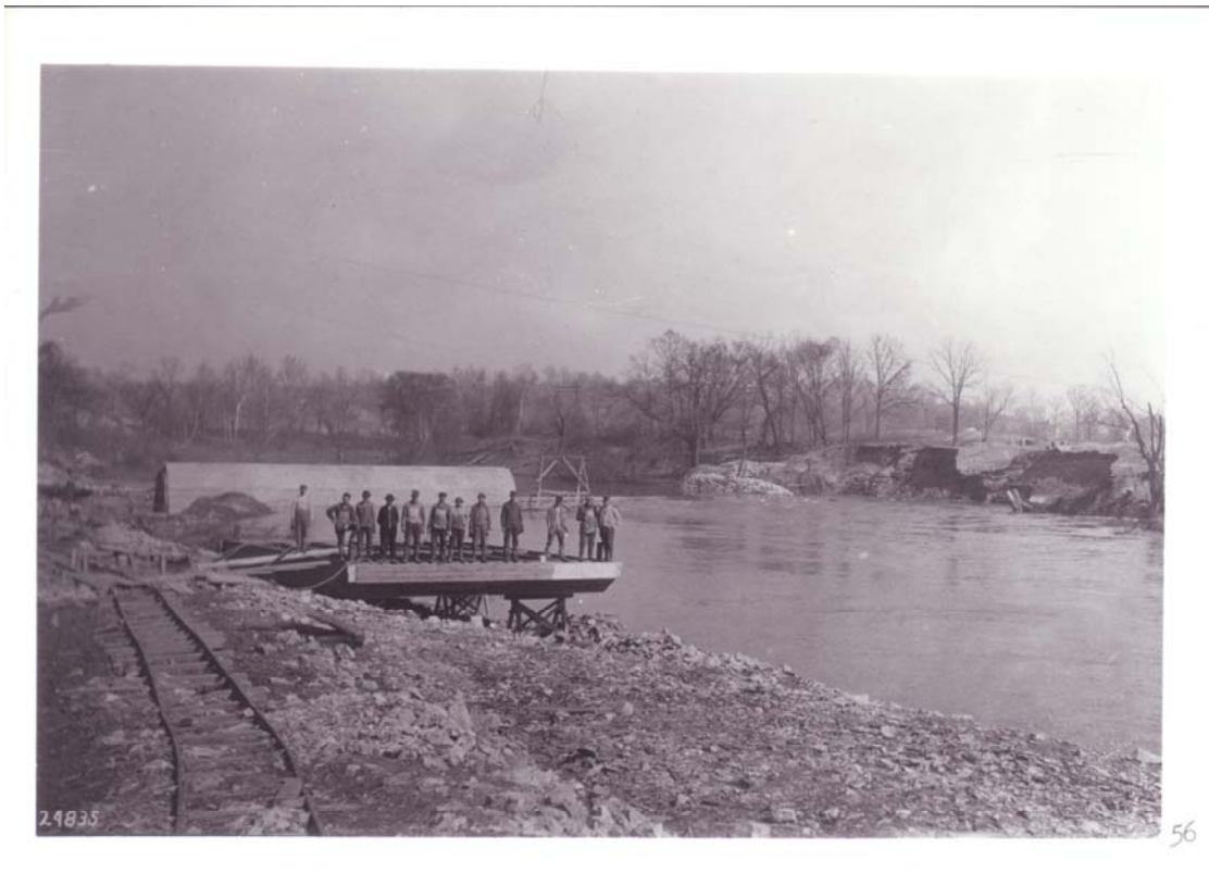
2/15/1911 – View of dam and pile driver boat.
