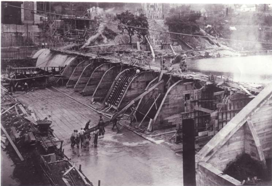
8/2/1911 – Concreting top of mattress, apron coating.
