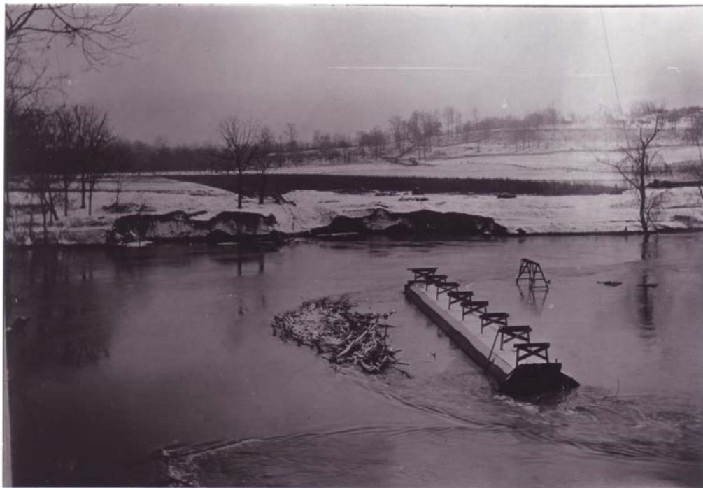
1/17/1911 – View of flood looking east from runway to mixer. Mixer removed.
