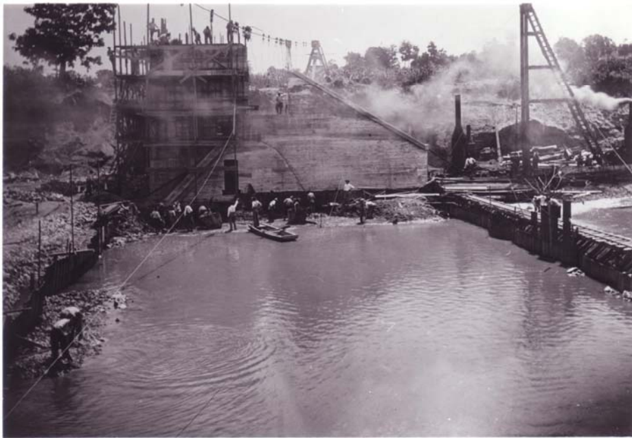
7/18/1911 – Excavation in east portion of dam from completed portion of dam.
