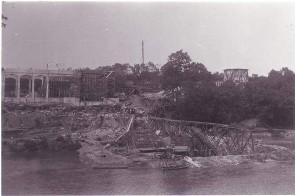
1910 – Williams Historic dam, construction photograph.
