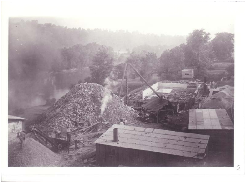
6/14/1910 – View from top of mill just north of site.
