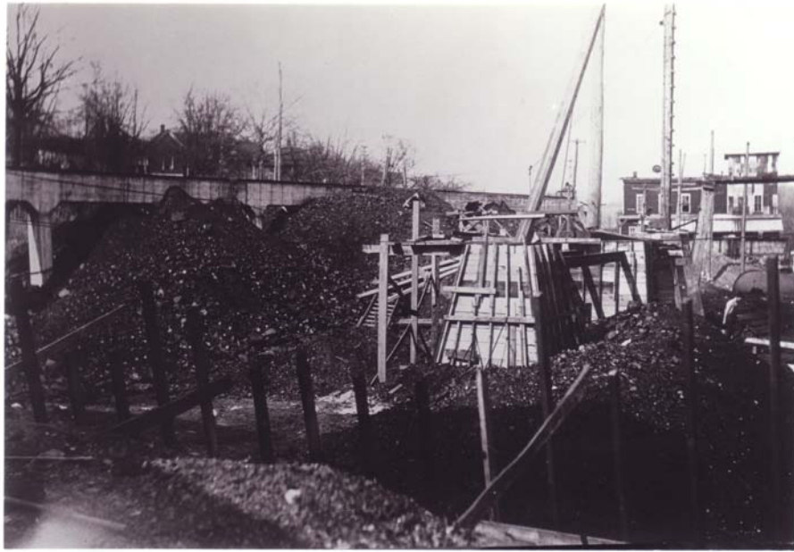
4/14/1912 – View of coal supply under trestle and coal derrick.
