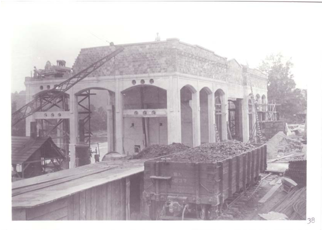
1910 – Williams Historic dam, construction photograph.
