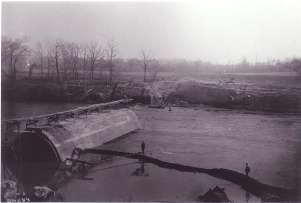
11/29/1910 – View of dam from boiler room level. Water over new coffer dam.
