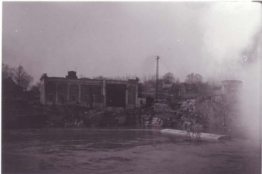
3/11/1911 – View of work and flood from opposite bank.
