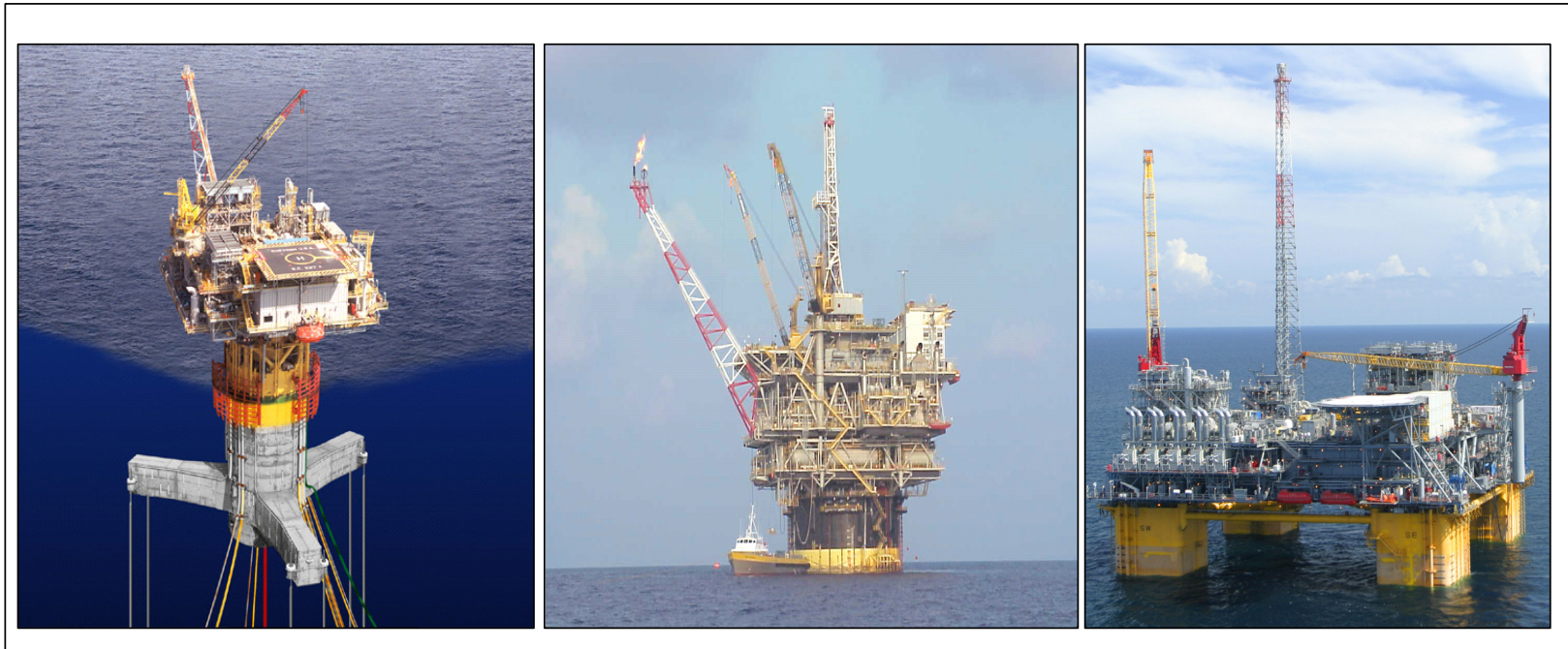
Figure 42. Three different development systems (left to right): a SeaStar TLP installed at ChevronTexaco's Typhoon field, a spar installed at ChevronTexaco's Genesis Field, and a semisubmersible at Shell/BP's Na Kika Field (images courtesy of ChevronTexaco, Shell International Exploration and Production Inc., and BP).
