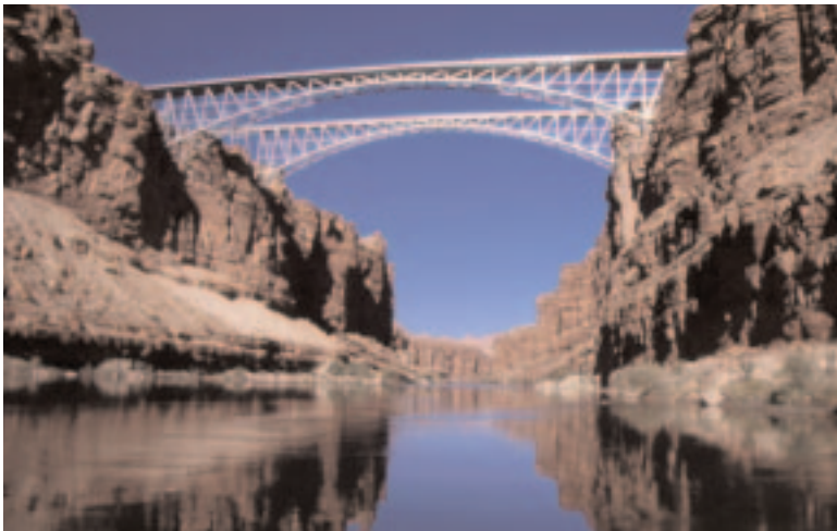
Navajo Bridge; US 89-A crossing the Colorado River at Marble Canyon, Coconino County
