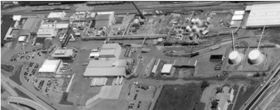
Photo: Rohm and Haas' Knoxville, TN plant
