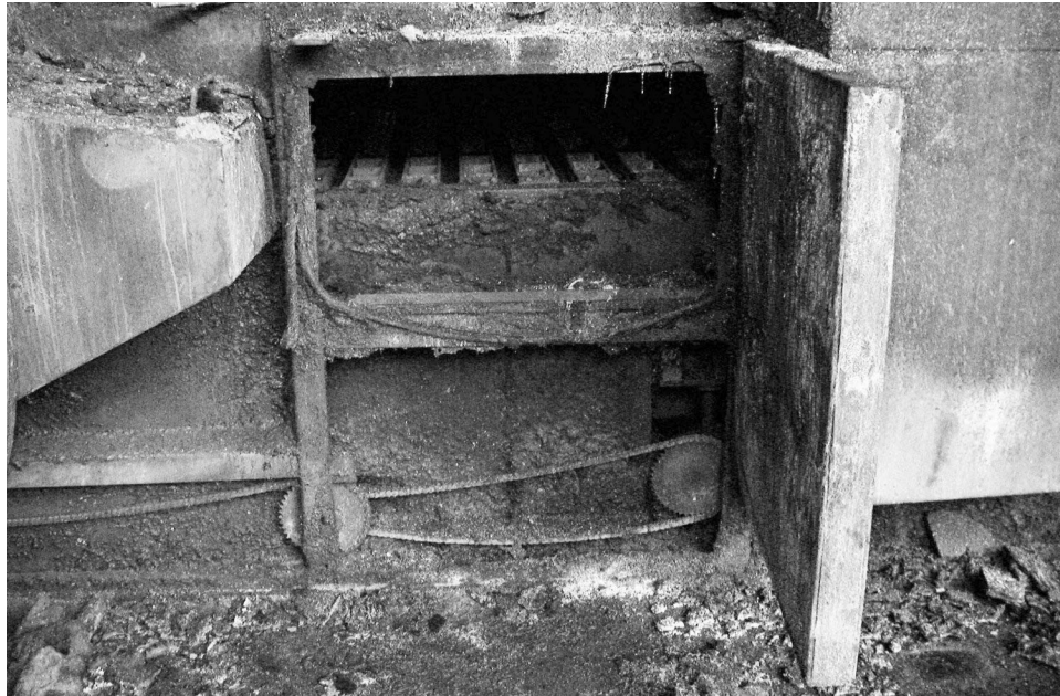
Figure 13. Interior of line 405 oven.
