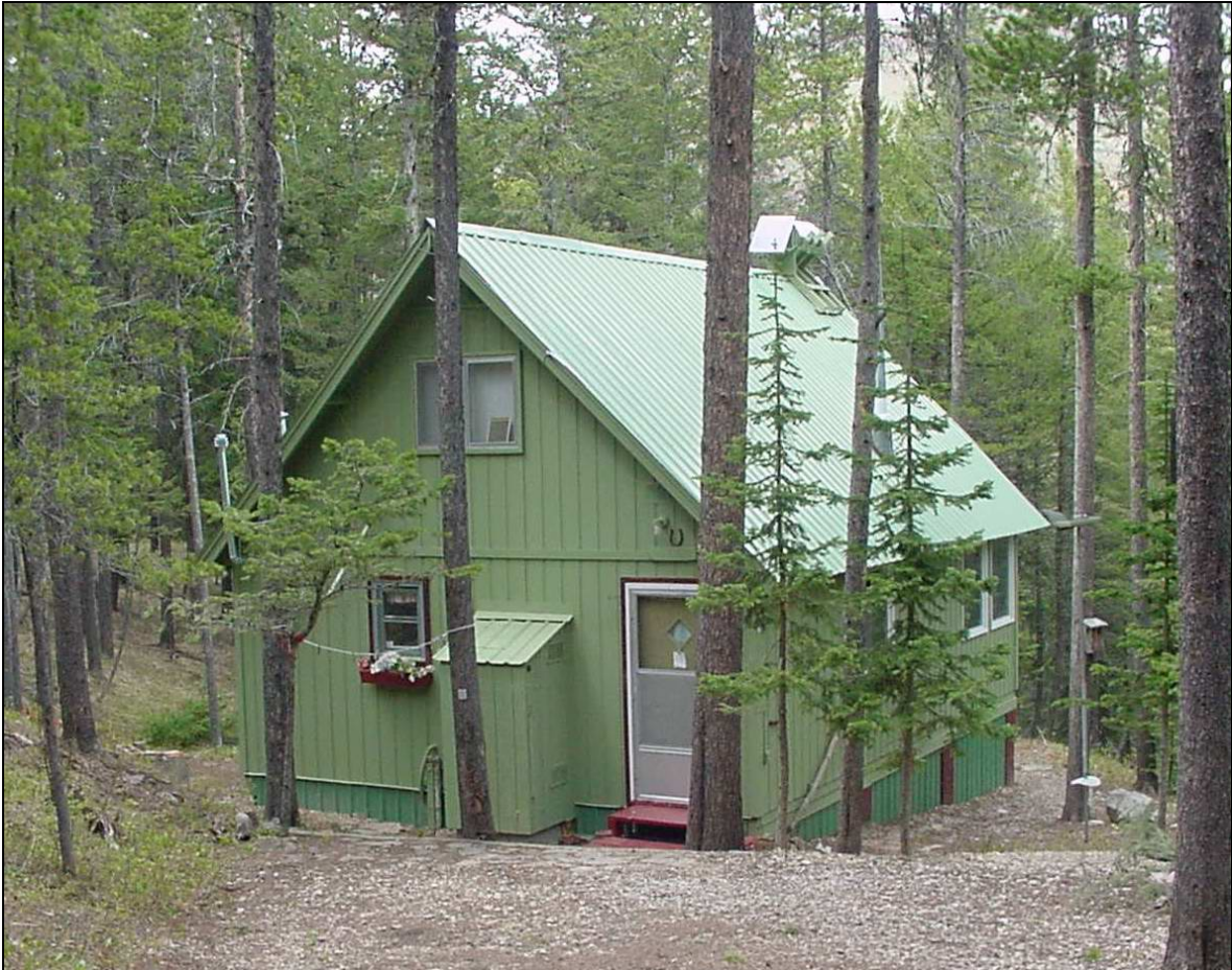
Figure 10. Group 4 rectangular-plan cabin with modified gable on Lewis and Clark National Forest.
