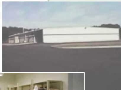
Bldg. 855 is used for the storage of site generated industrial, hazardous and Polychlorinated Biphenyl (PCB) solid, liquid, and gaseous wastes. This building was designed and built to provide tertiary containment for stored wastes to prevent environmental contamination should a spill occur. This was accomplished through the use of sealed concrete and an impervious liner placed under the building that exceeds regulatory requirements.
