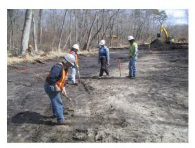
One of the pictures that Skip showed to the working group: Taken on March 9, the picture shows workers reconstructing the river channel following excavation of sediment. In the background, an excavator continues removing contaminated sediment from the central stockpile.
