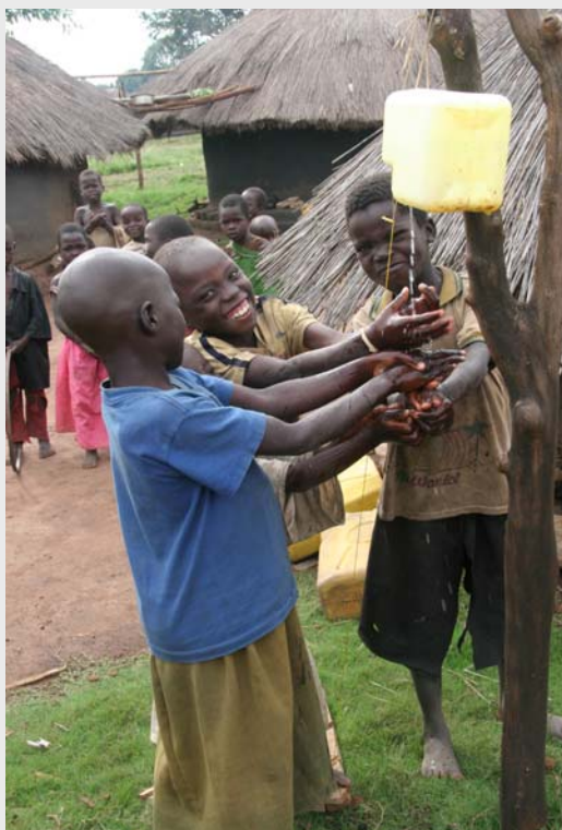
Children in Pader Camp use hand washing sites installed with OFDA funds (Jack Myer, USAID).
