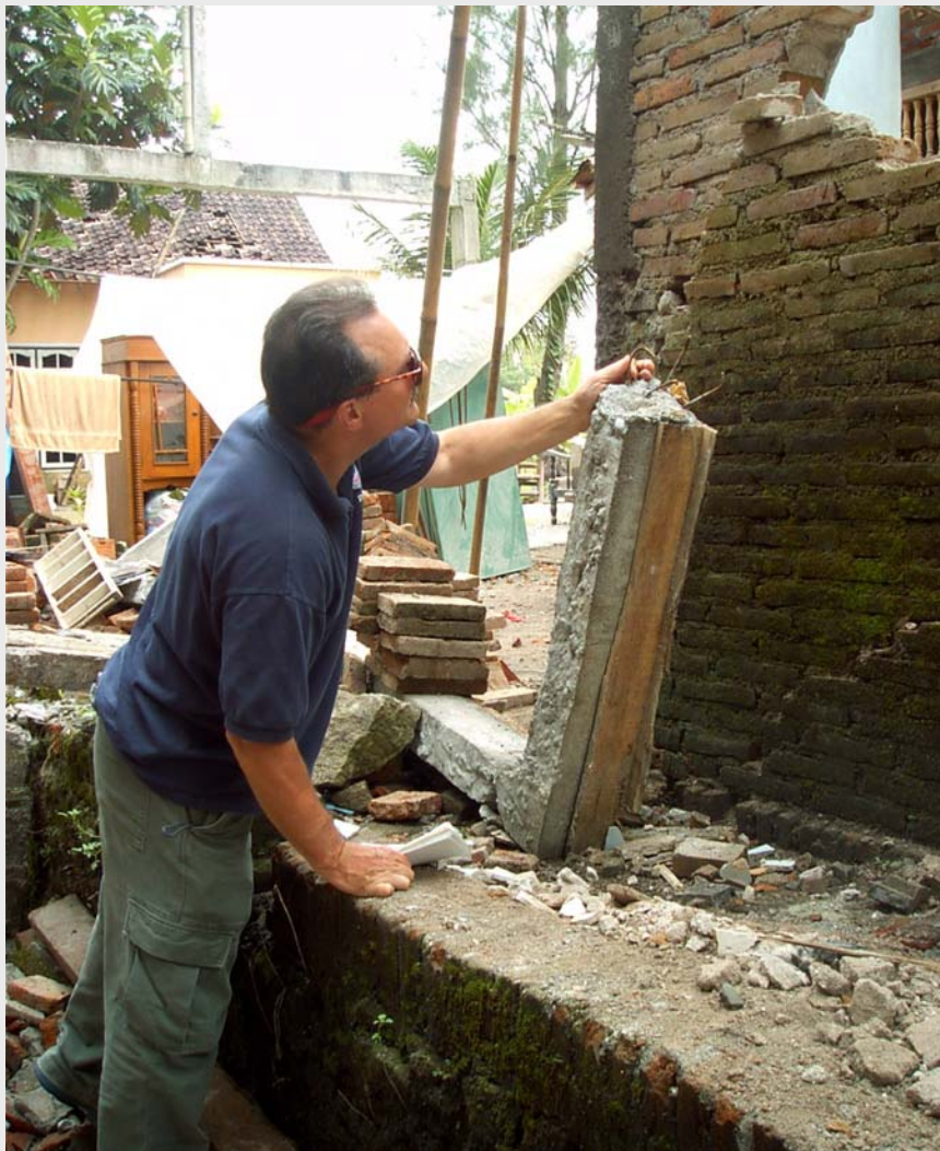
An OFDA shelter specialist examines earthquake-damaged buildings in Indonesia (Alfred Nakatsuma, USAID).
