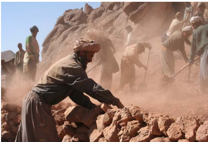
Afghanis build roads through OFDA-funded cash-for-work programs (CRS).
