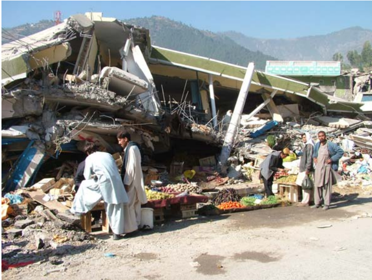
A street market reopens in the shadow of earthquake-damaged buildings in Batagram, Pakistan (USAID/Pakistan).
