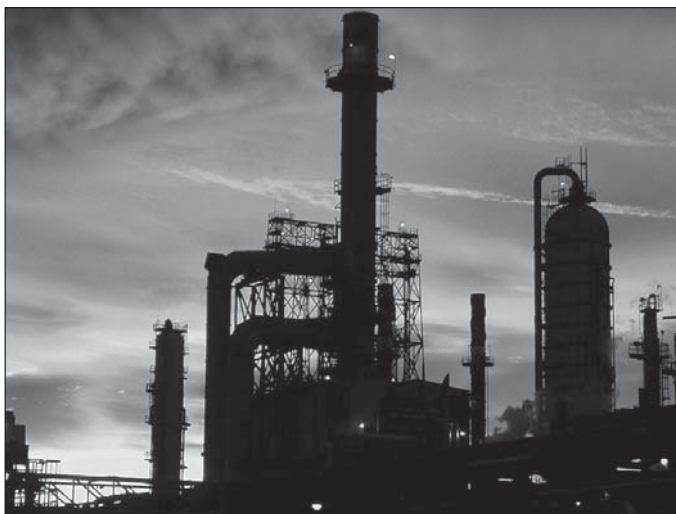
C3's "super ceramic" coatings are being studied to see if they could help petrochemical plants reduce carbon dioxide emissions.
