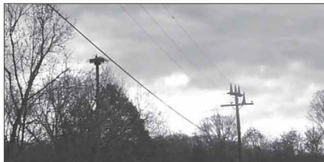
A nesting osprey on an artificial platform is on the left, and a power pole that's been "discouraged" is on the right, in the 0800 area.
