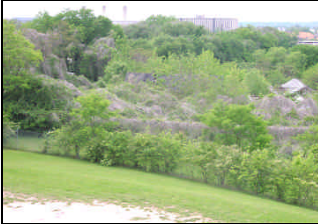
Photo 1: Overview of the southern portion of the former AOC and NRS areas of the Site, facing northwest (from the Anacostia Station parking structure photographed on May 6, 2002).
