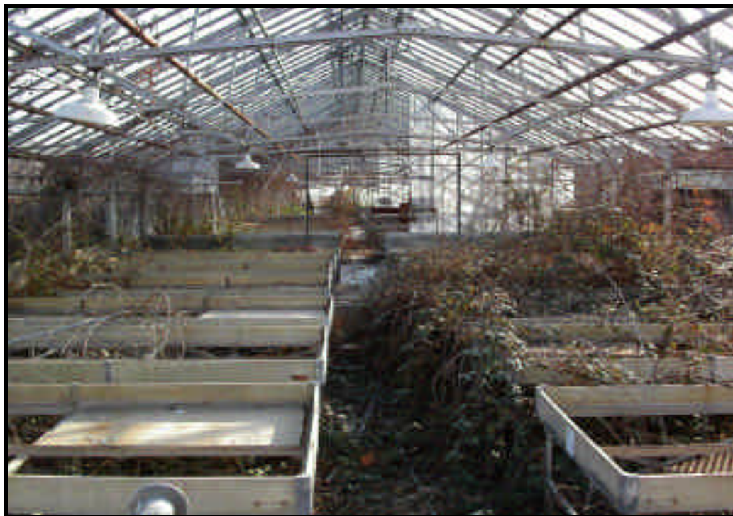
Photo 6: Interior of easternmost northern greenhouse (photographed on December 18, 2002).
