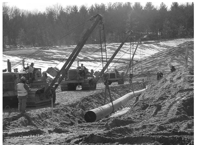
Pipelayers lay clay, concrete, plastic, or cast-iron pipe for drains, sewers, water mains, and oil or gas lines.
