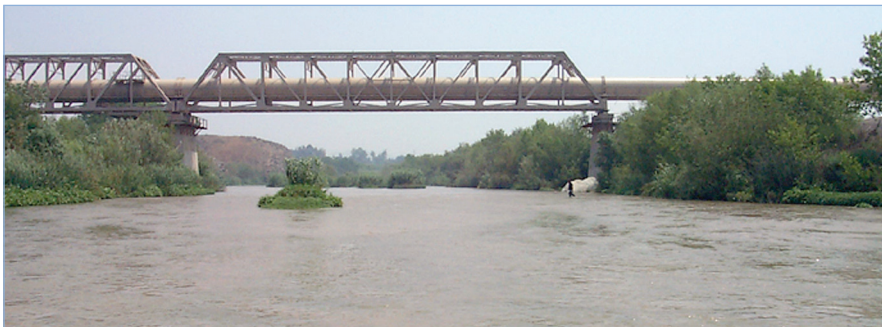
Santa Ana River at MWD Crossing. Pipeline conveys imported surface-water deliveries. (photograph by Carmen Burton, U.S. Geological Survey)
