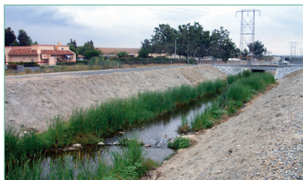
Little Chino Creek is one of many tributaries that have been channelized for flood control. (photograph by Carmen Burton, U.S. Geological Survey)
