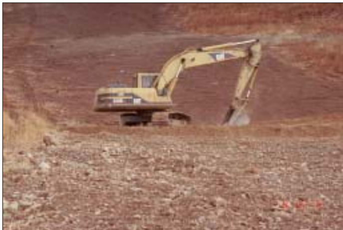
Waterbar installation by trackhoe excavator.
