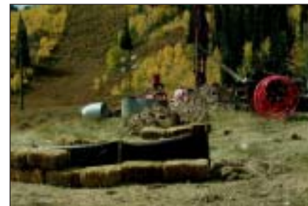
Accidental spillage of drilling fluids should be well contained and filtered before entering streams.
