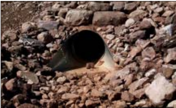
Oversized culverts on steep gradient channels allow passage of large channel substrate rocks.
