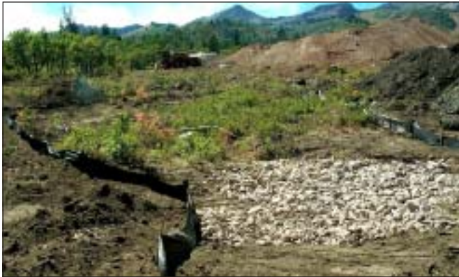
Sediment fencing can be used to define subtle drainage areas and protect them from sediment as well as unauthorized vehicle traffic.
