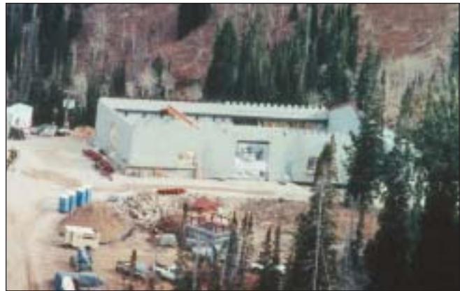
Stockpiles from foundation excavations should be contained within sediment trapping barriers.
