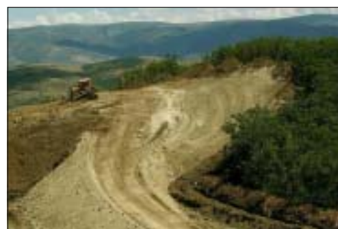
For ease of reapplication, topsoil can be stockpiled in windrows at the top of steep slopes.
