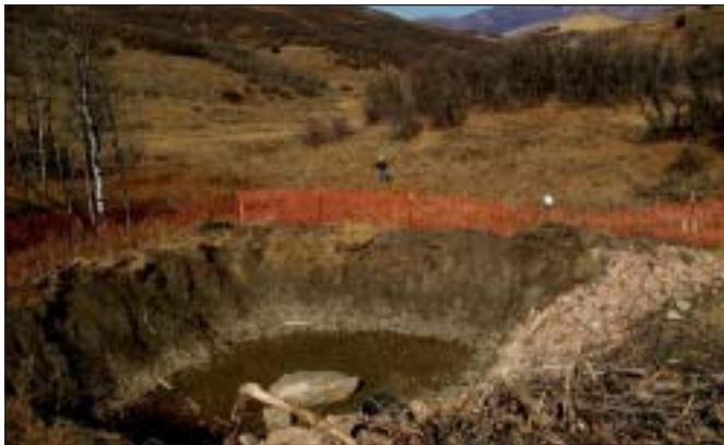
Use detention basins to capture sediment before it can reach wetlands and riparian areas.
