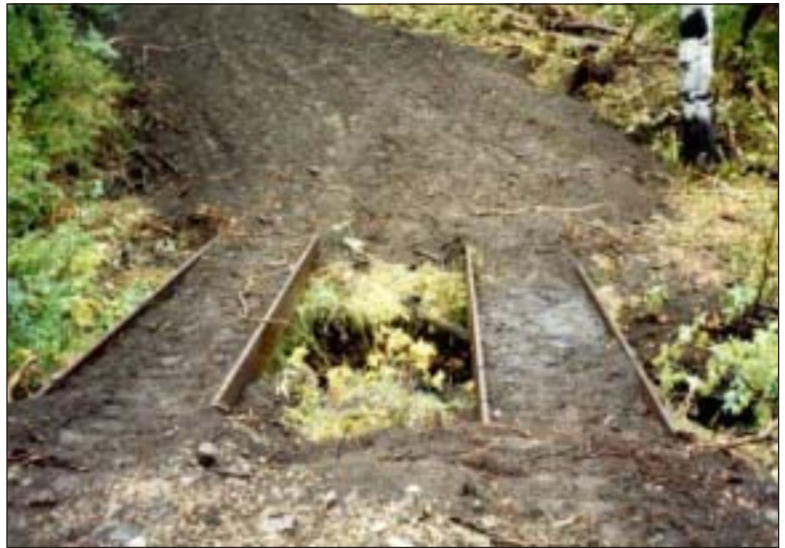
Temporary bridging methods allow for heavy equipment to cross streams with minimal disturbance to channels.
