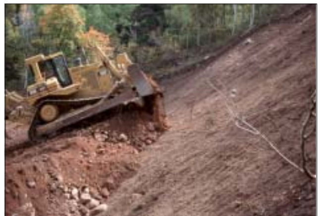
Swales and slope break compressions can be smoothed out by filling with subsoil excavated from building and lift terminal foundations.
