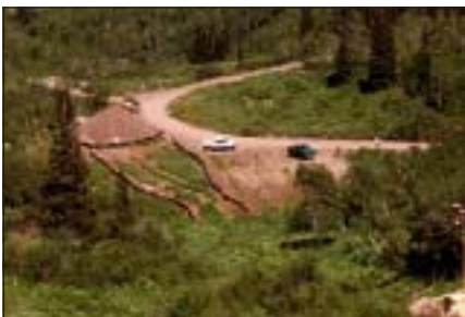
Water from well production tests should be filtered of sediments prior to discharge into wetlands.
