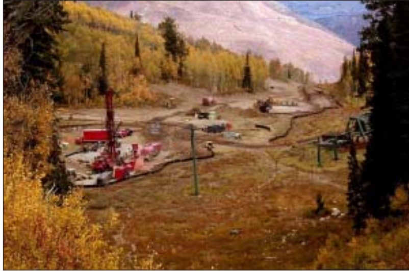
Backslope and drain well pads away from nearby streams and wetlands.
