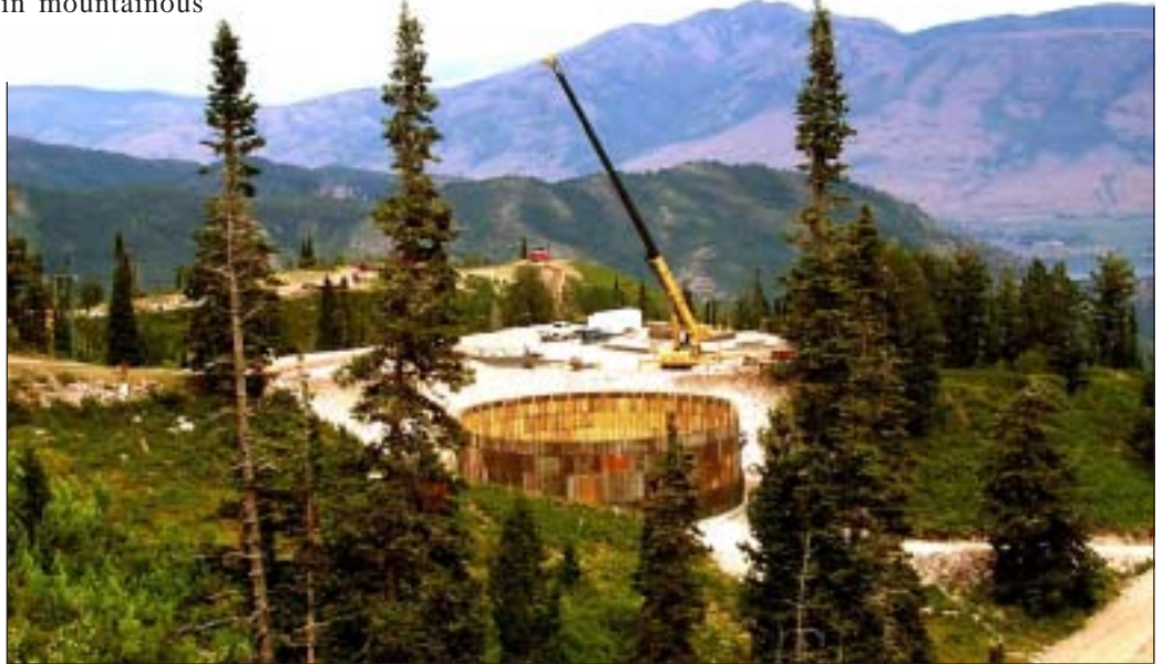
Staging areas and access roads can be built from storage tank excavation material.
