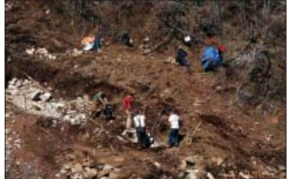
Tower foundations in steep or remote terrain may require excavation by hand crews.
