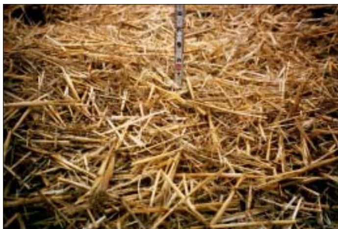
Straw mulch should be applied at a loose thickness of four to six inches.
