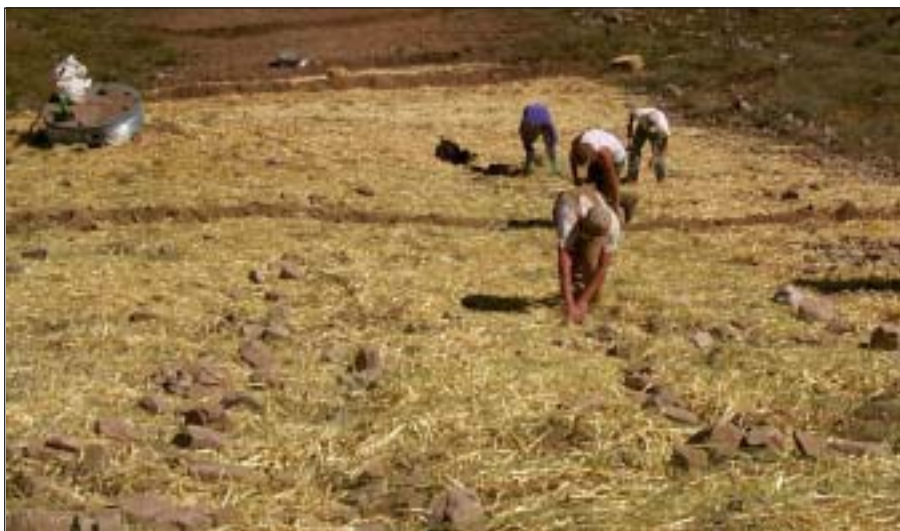
Straw mulches cannot be tracked into rocky or dry soils, and must be secured with either netting or chemical tackifiers.
