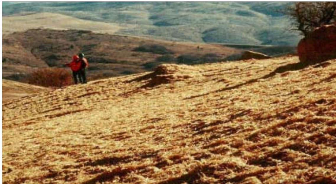
When properly tracked in, straw will be punched into the soil and appear to stand upright.
