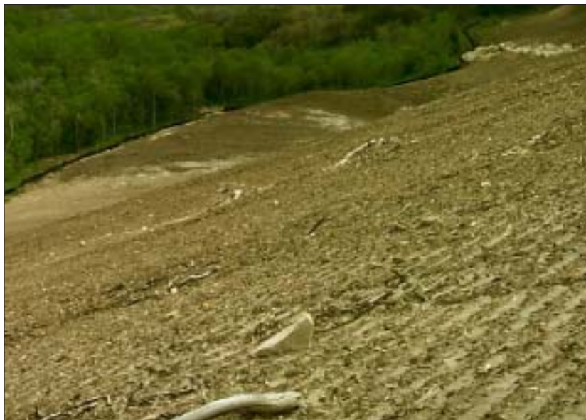
The final reclaimed surface can be roughened with bull dozer tracks to provide micro-sites for moisture conservation and seedling establishment.
