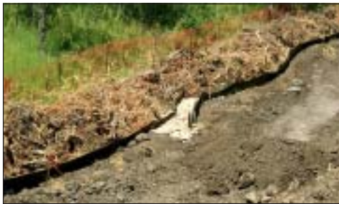
Cleared vegetation can also be used as a filter by placing and compacting into a windrow.
