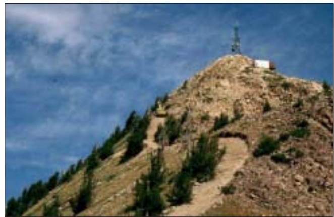
Snow cat access trails can be constructed to narrower widths and then widened with snow.
