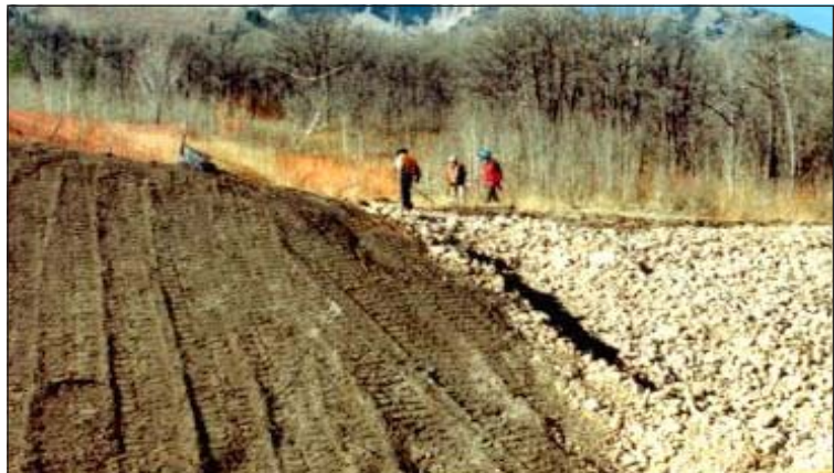
The most important disturbed land reclamation task is to restore a thick layer of fertile topsoil.
