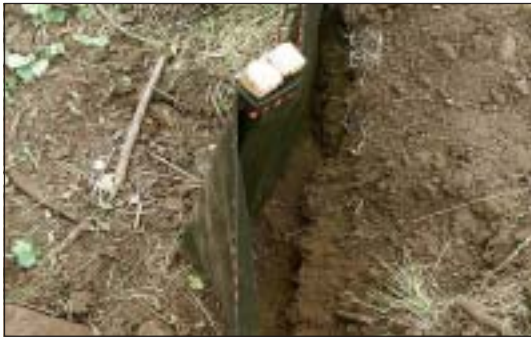
Fencing can be lengthened by wrapping section ends together and then securing tightly with wire.
