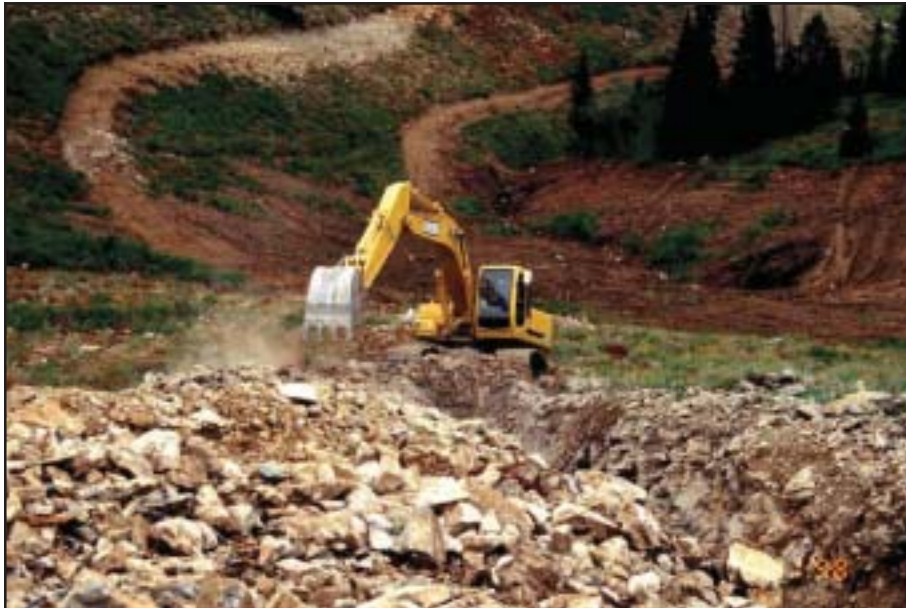
Topsoil is a scarce resource in many mountain environments. Trench excavation should salvage topsoil where present to use in restoration work.
