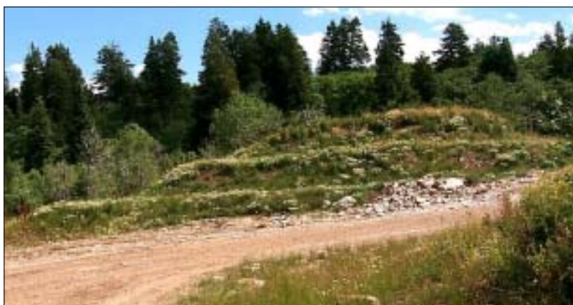
If stored over the winter, topsoil stockpiles should be terraced and seeded to reduce erosion losses and should then be surrounded with sediment control measures such as berms, silt fencing, or straw bale dikes.
