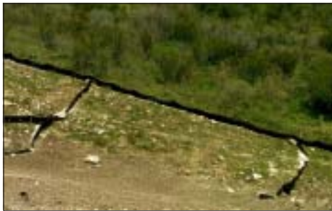
A stream side riparian zone may also be used to filter out finer sediments which can pass right through sediment fencing.
