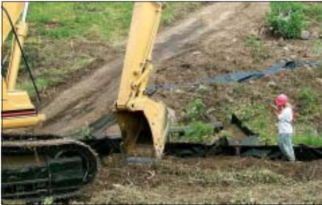
An excavator is useful in silt fence installation. Fencing should be placed in pre-dug trenches, and backfilled to prevent breaching under the fence bottom.
