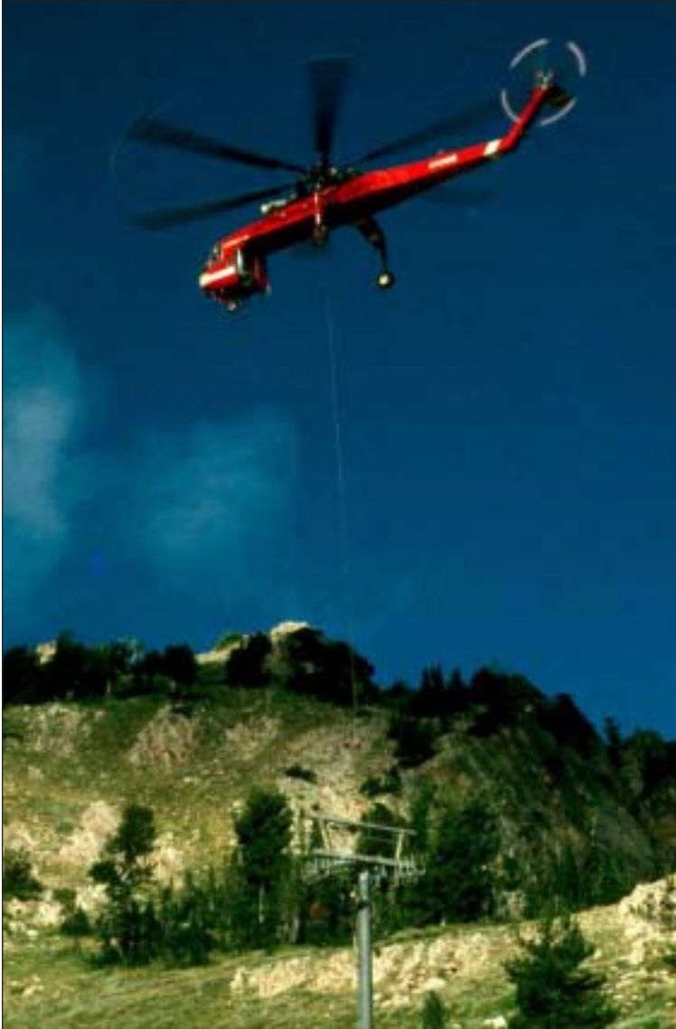
Towers and cable gantries can be lifted and placed in remote locations with large helicopter sky cranes.
