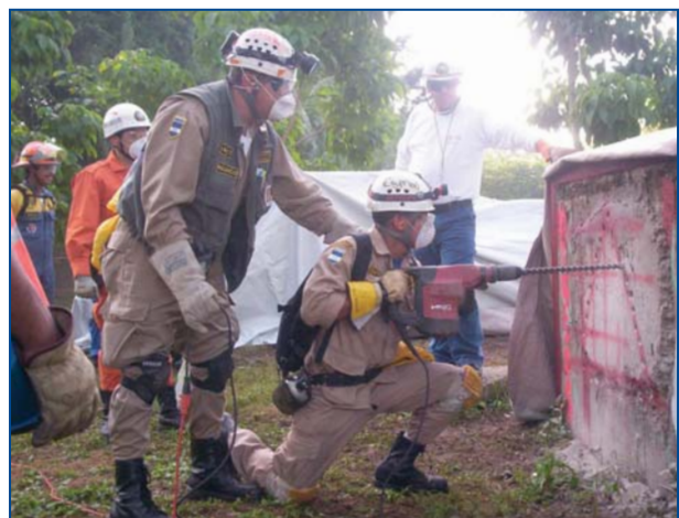
Teams practice penetrating collapsed structures as part of OFDA's Search and Rescue of Collapsed Structures (BREC) course.
