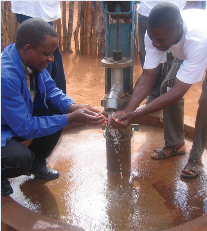
Beneficiaries enjoy clean water from a well constructed with support from OFDA in Zimbabwe.
