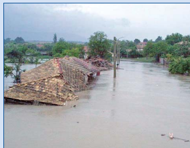
Floodwaters engulf houses in Bulgaria.
