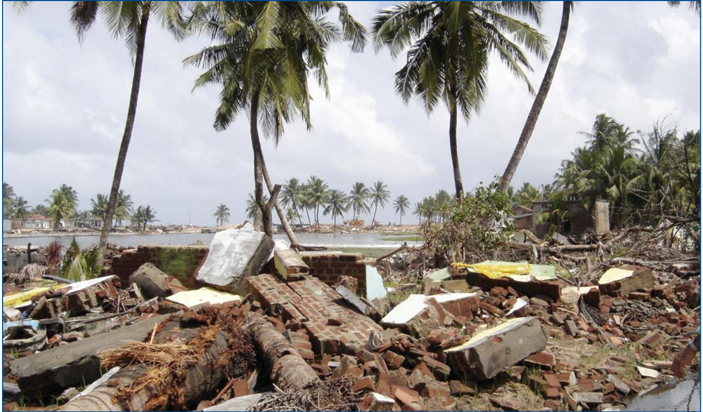
The impact of the tsunami leaves structures along the coast of Ampara, Sri Lanka, in ruins.
