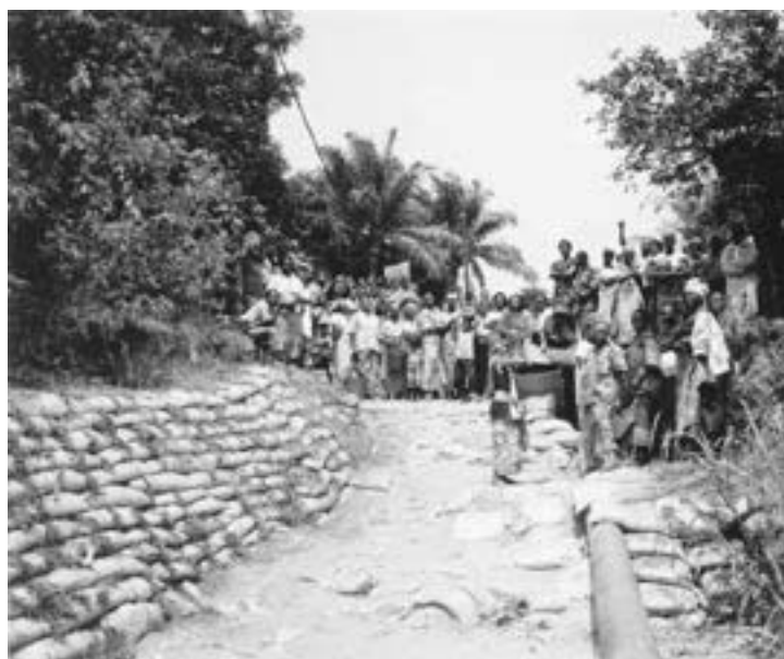
Residents of Kinshasa gather to inspect newly reinforced embankments of a neighboring river as part of a USAID/OFDA-funded flood mitigation project (photo by Marion Pratt, USAID/OFDA).
