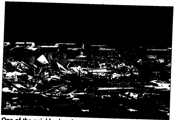
One of the neighborhoods seriously damaged by Hurricane Luis.
