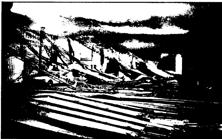
The World Food Program warehouse in Nacala collapsed as a result of 90 mile-per-hour winds from Cyclone Nadia. (Photo by Kevin Carlson, USAID/Maputo)
