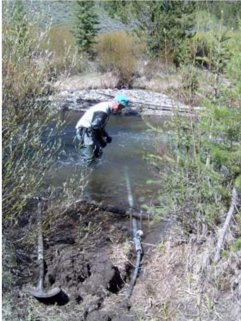
Gage installation at Fourth of July Creek near Stanley, Idaho
