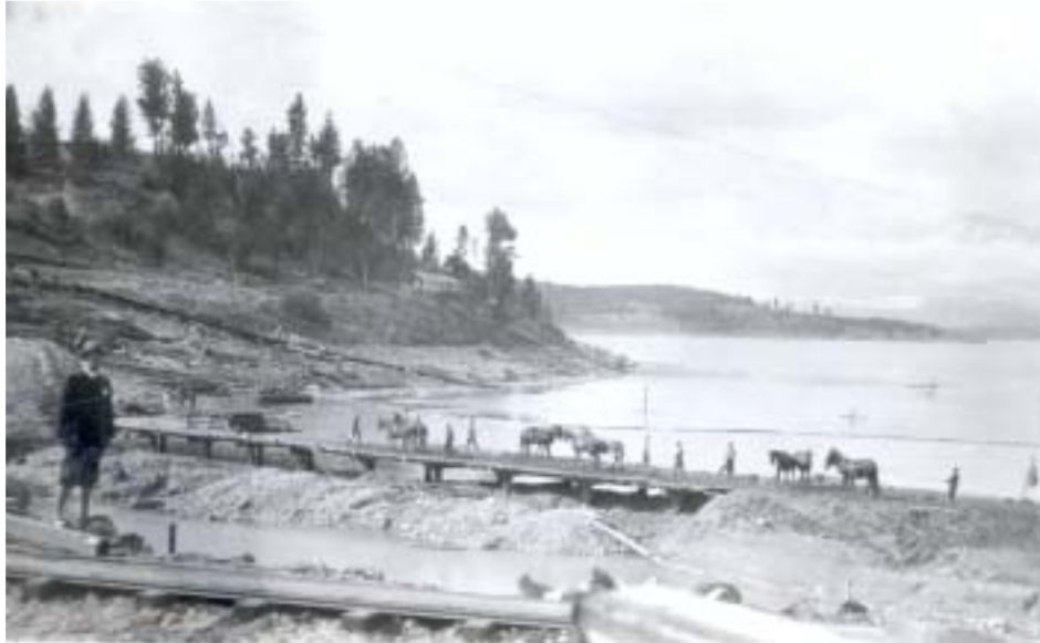
Construction work on Jackson Lake dam, Upper Snake River basin (Oct. 1914)
