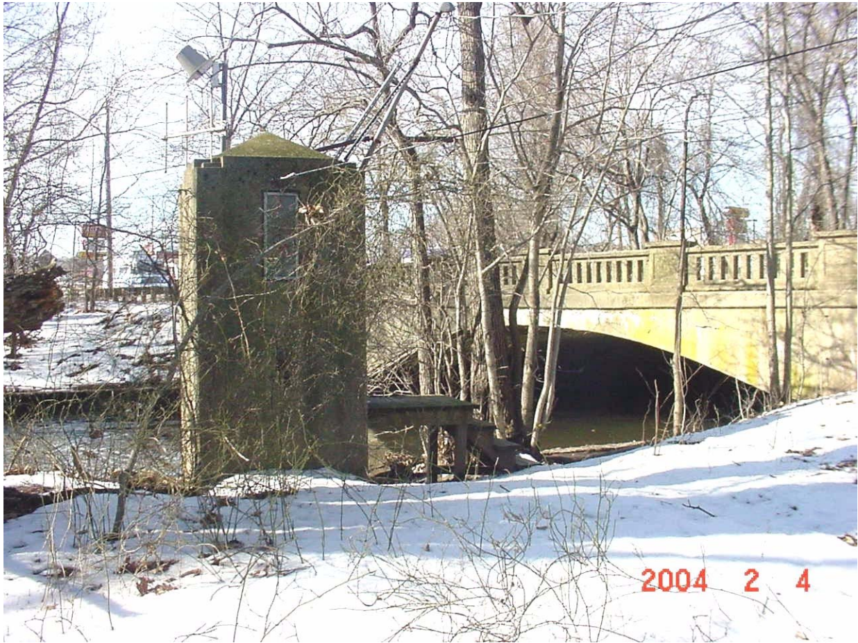
Figure 16. U.S. Geological Survey gage continuously monitoring the stage of the Rahway River near Springfield, NJ. Photograph taken by Blaine White, 2004.
