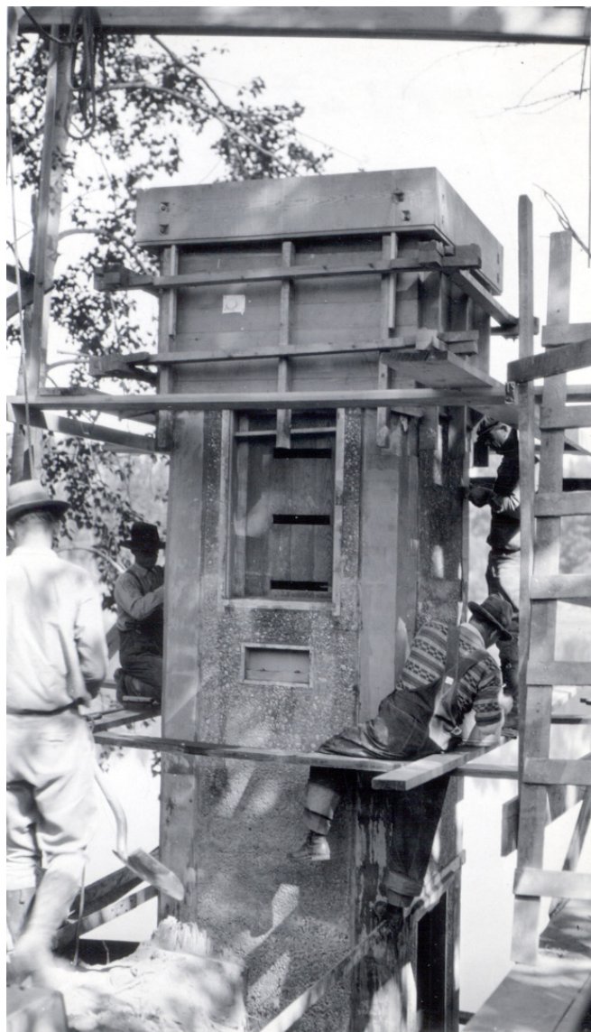
Building the Kootenai River at Porthill gage house.
