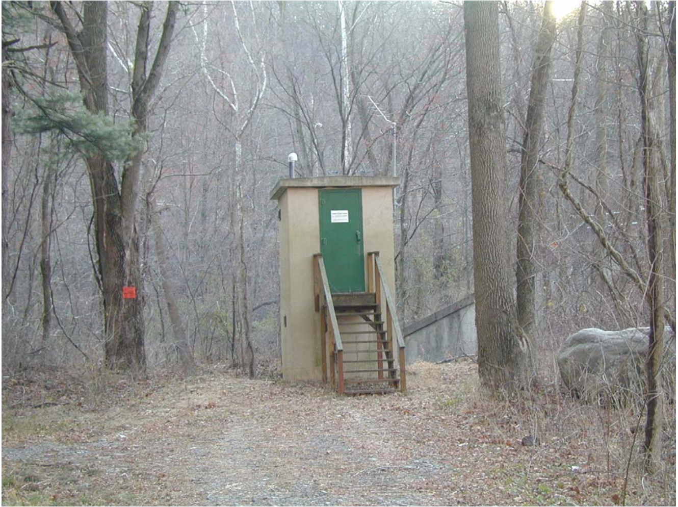
Figure 14. U.S. Geological Survey gage continuously monitoring the stage of the Pequannock River at Macopin Intake Dam, NJ. Photograph taken by Rick Edwards, 2002
