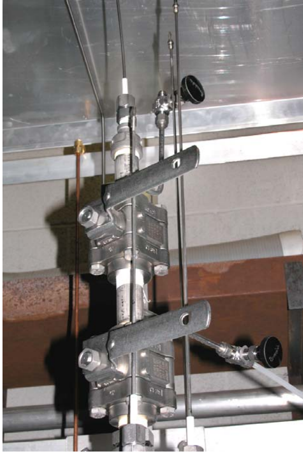
Fig. 2. Assembly at top of surge tank showing double ball valve for salt sampling and three electrodes for cyclic voltammetry.
