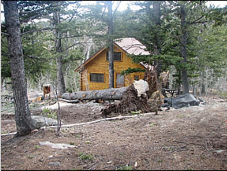
Photo 4: A Douglas-fir that reportedly fell during Monday’s wind event, a short distance from the fire. Photo by Clint Dawson, Shoshone NF.
