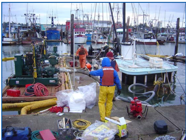
Pumping out the vessel
