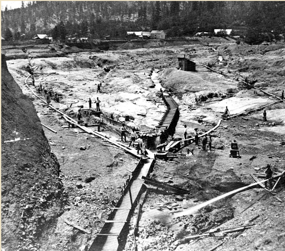
Figure 21. Gravel deposits were washed into sluices where gold was recovered by gravity separation. Amalgamation with elemental mercury was then used to extract the gold (about 1850). (Photograph courtesy of Siskiyou County Historical Society.)
