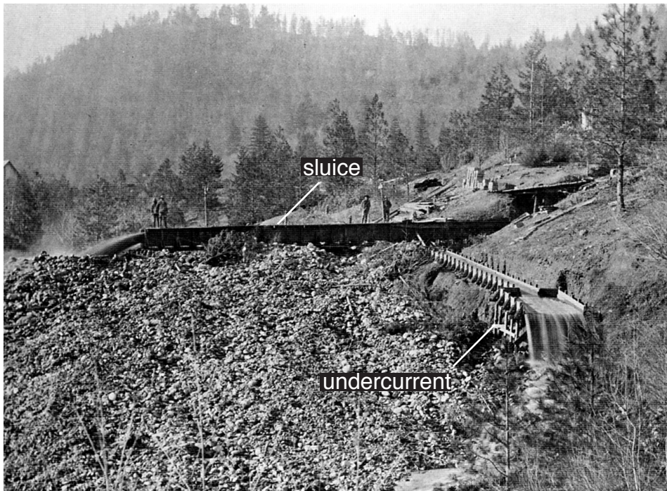
Figure 23. View of sluice system, Siskiyou County, California (about 1860). (Photograph courtesy of Siskiyou County Historical Society.)
