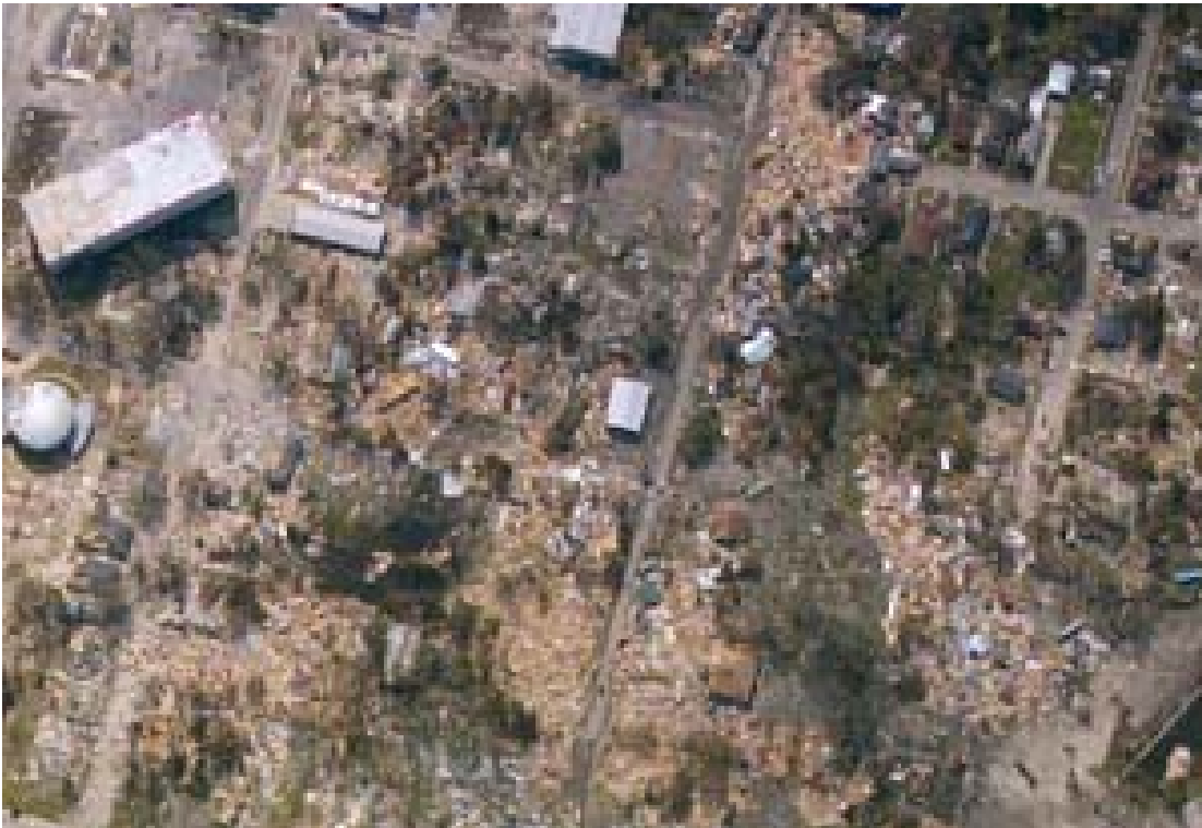
Picture 2. Damage in Ocean Springs, MS. Photo taken by NOAA on August 30, 2005.
