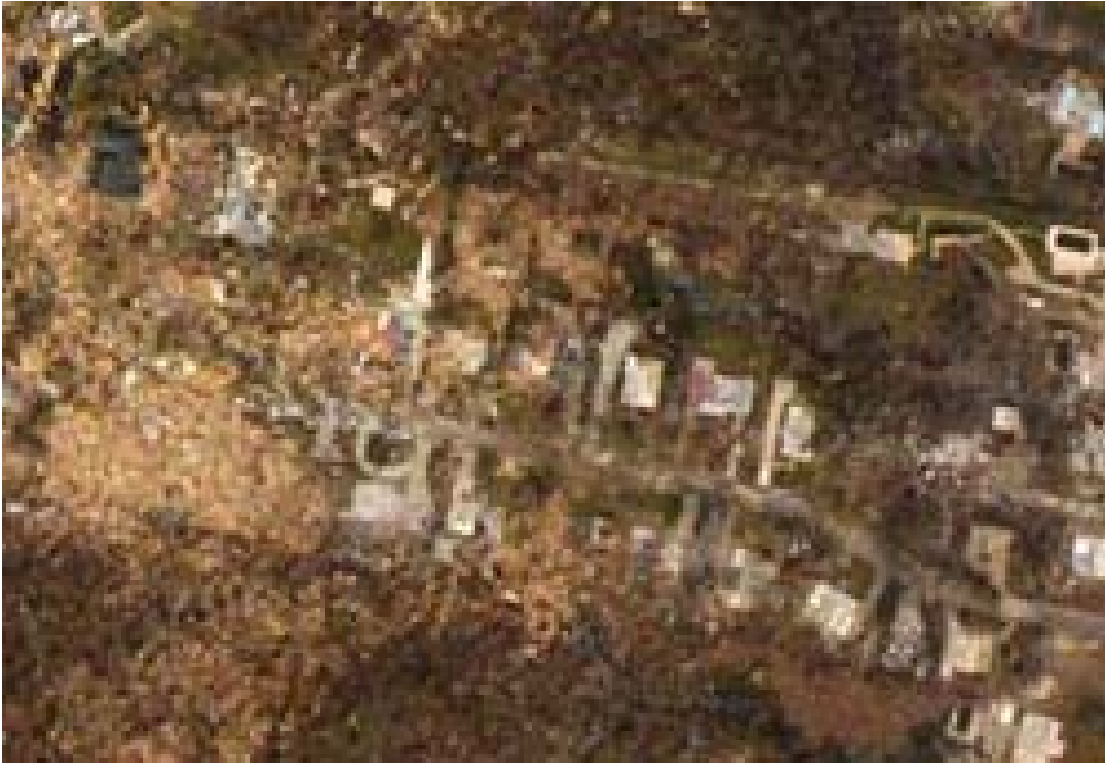
Picture 3. Damage from Bay St. Louis, MS. Photo taken by NOAA on August 30, 2005.
