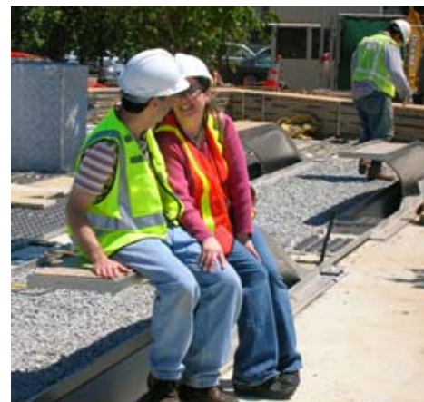
The focus of the memorial are the 184 cantilevered benches built over a pools of lighted water. US Forest Service photo by Leslie Weldon. Click to enlarge.
