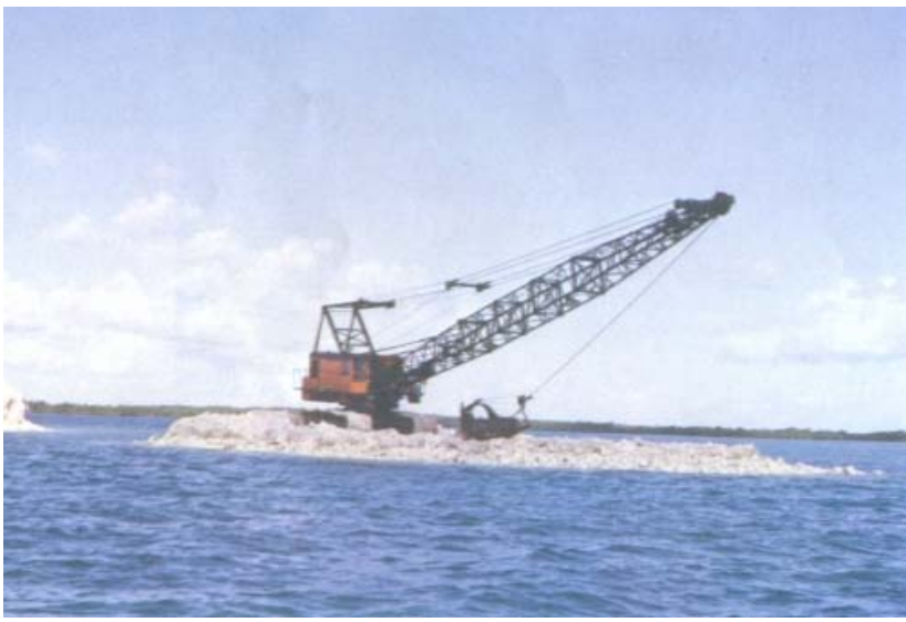
Dredging of coral.
