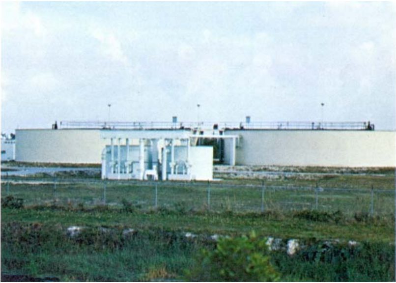
Twenty-nine sewage treatment plants serve the south Dade area.
