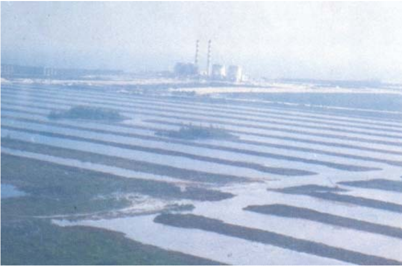
More than 10 miles of cooling canals have been constructed at the Turkey Point power plant to cool the circulating water. (Photo by Penny Zobel)
