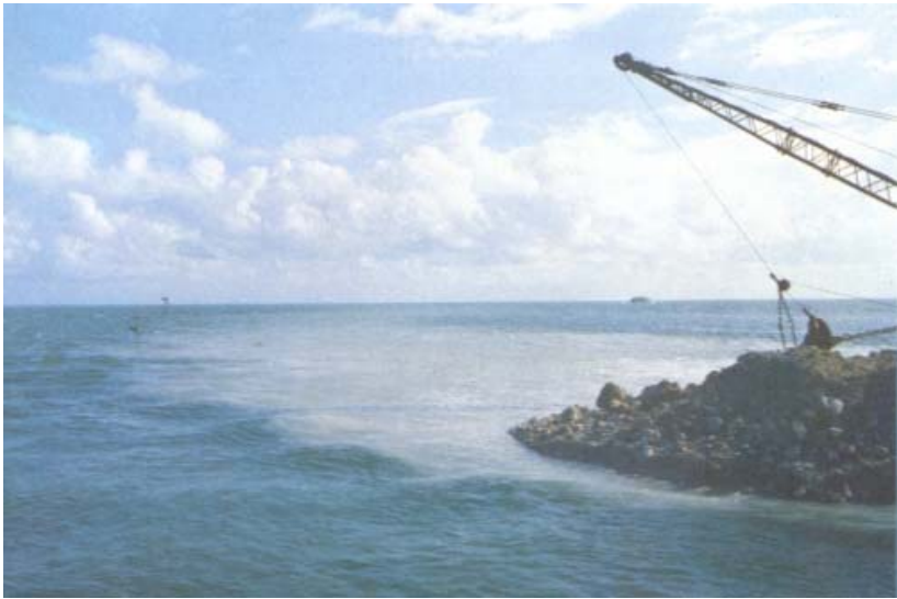
Silt from turbid or muddy waters caused by dredge and fill operations smothers and kills coral reefs.
