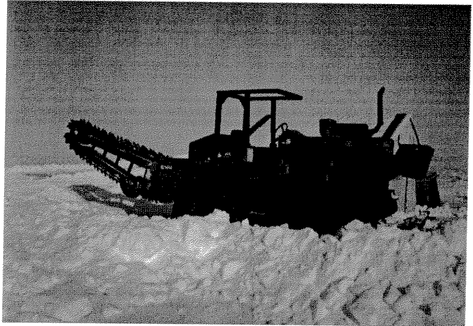
Fig. 8 R-100 DitchWitch used for Phase 2
