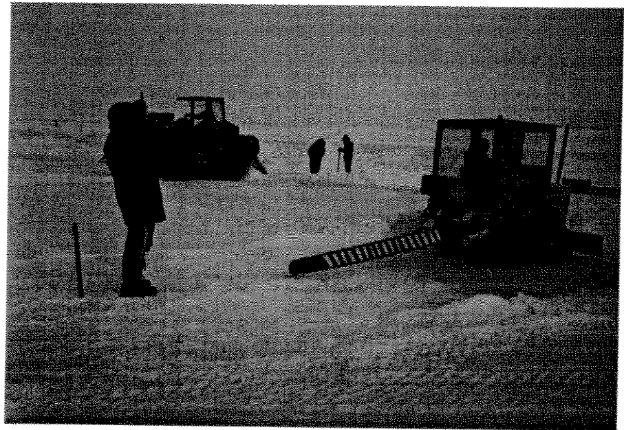
Fig. 9 Lining up NRC Ditch Witch to cut the pre-crack
