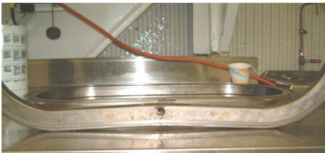
Another view of the crushed door seal carrier, illustrating the amount of damage caused to the seal. The single fastener in the center of the seal sheared due to the force exerted by hydrostatic pressure
