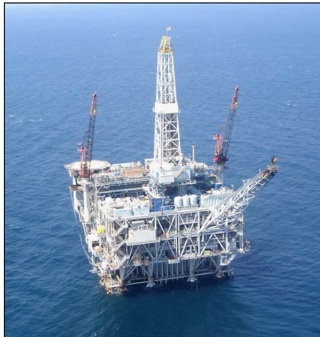
Figure 7. Open structure with large amount of small diameter bracing, such as found with jackups (top), have the potential to allow large superstructure icing loads. The Heritage rig, (bottom) located off of the Santa Barbara coast, would have serious icing problems with its complex structure if operated in cold waters.
