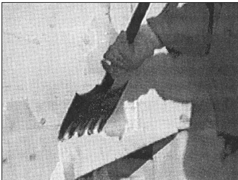
Figure 44. Five-point chisel in use by Chief on CGC Midgett , 1990.
