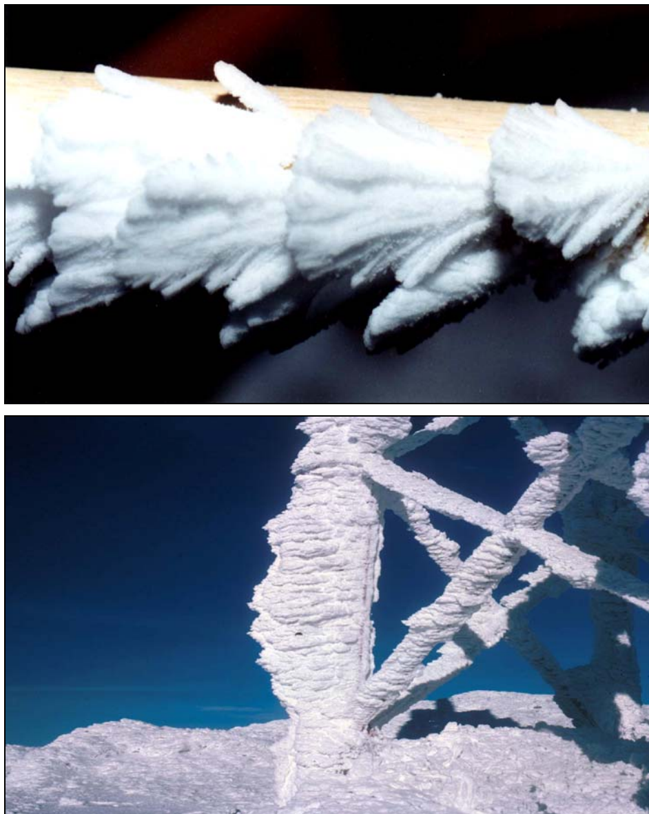
Figure 2. Supercooled cloud drops freeze quickly, trapping air. They form rime feathers on the upwind sides of objects (top) and can form deposits more than a meter thick on towers (bottom).
