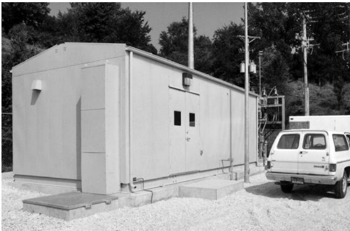
Figure 16-1: Pre-Engineered Metal Control Building (Coffeyville, KS)
