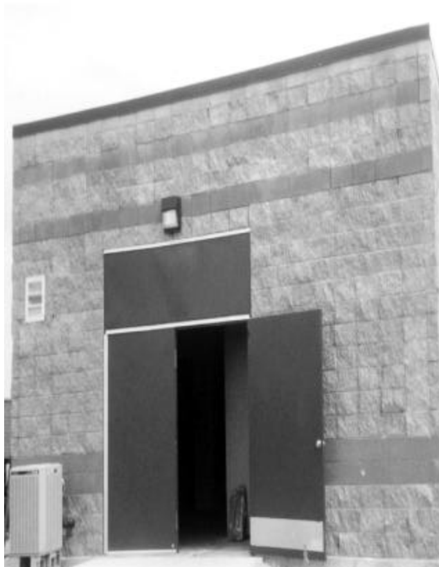
Figure 16-3: Architecturally-Pleasing Masonry Building (Rochelle)
