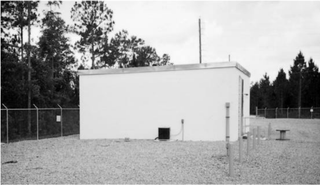
Figure 16-2: Typical Masonry Block Control Building
