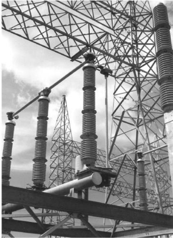
Figure 5-22: Horizontally Mounted Double Break Switch with Grounding Switch. Courtesy of Tuley & Associates, Inc.
