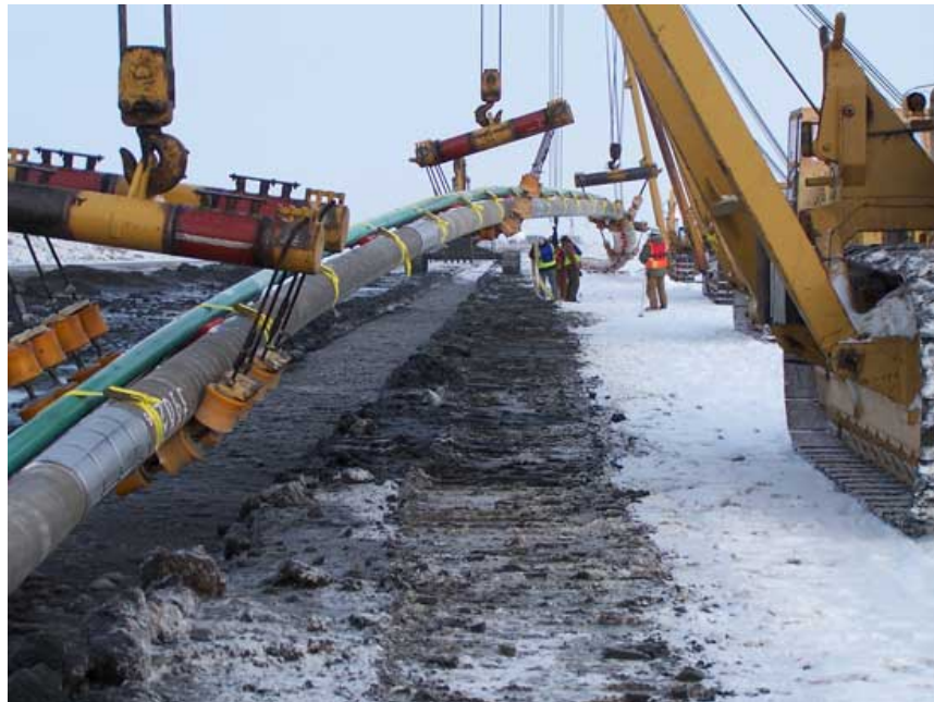
Figure 10-3: Through-ice installation of the Oooguruk pipeline bundle (H.C. Price Co., 2008)
