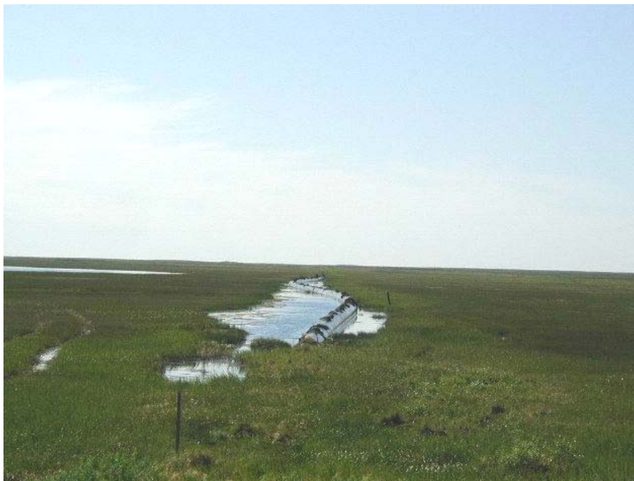
Figure 1-6: Example of onshore lateral buckling
