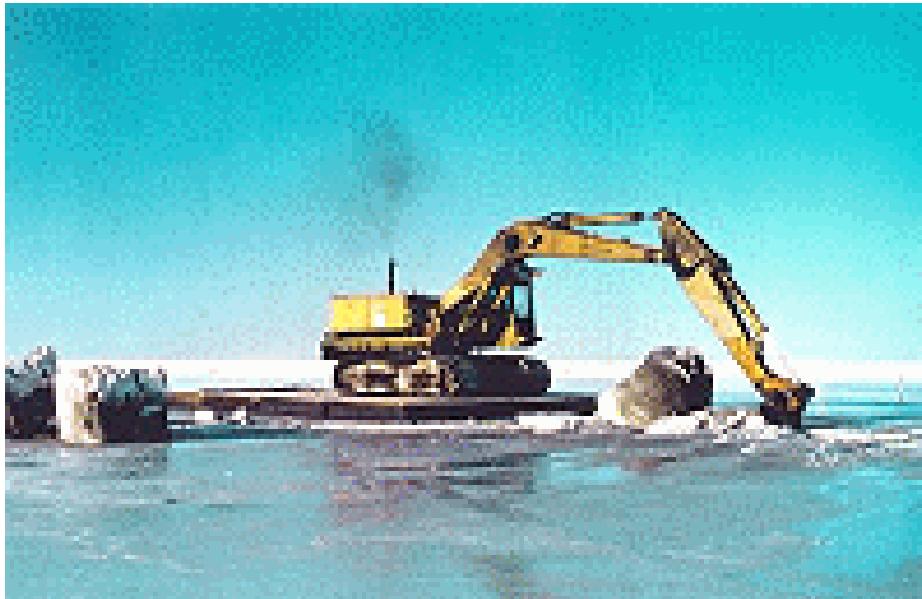
Figure 10-1: Northstar on-ice trench excavation trials (INTEC, 2006)
