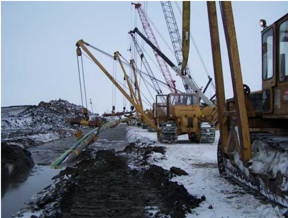
Figure 10-4: Through-ice installation of the Oooguruk pipeline bundle (H.C. Price Co., 2008)
