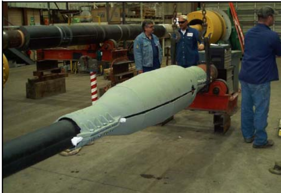
Figure 4.4: Shroud Installed on TSJ (Credit: RTI Energy Systems)
