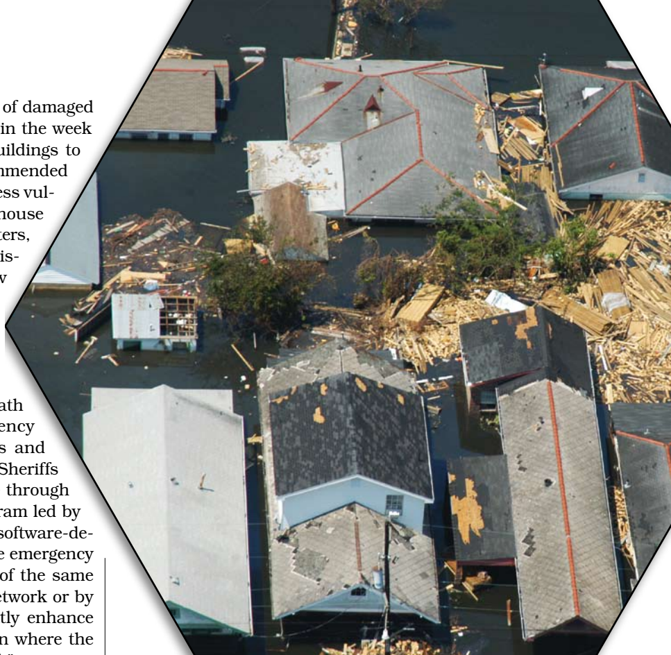
New Orleans roofs damaged by Hurricane Katrina
