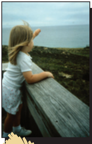
Figure 80—Caution: railings with horizontal rails make an inviting ladder for small children.
