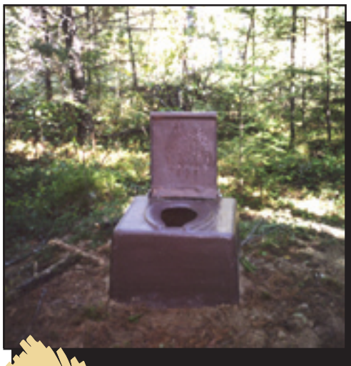
Figure 84—A fiberglass riser for a pit toilet in the Boundary Waters Canoe Area.
