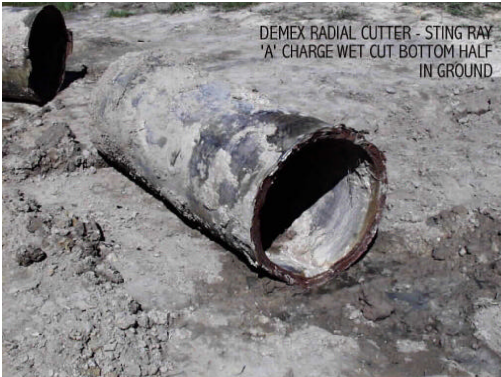
Photo 17. Inside Shaped Charge Cut on 26'' x 1.25'' wall pile
