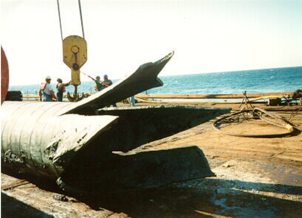
Photo 18. Bulk Charge Cut on 48" x 2" wall pile
