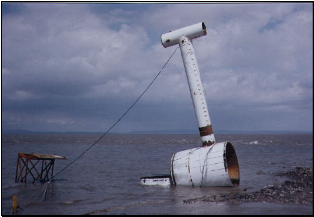
Photo 32. Resultant Cut of Structure
