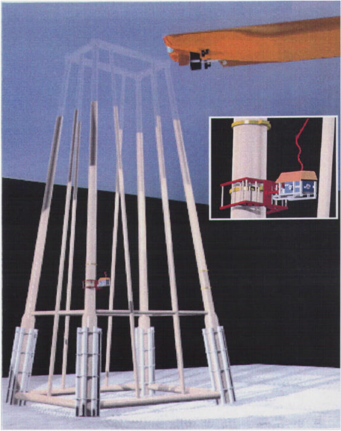
Figure 33. Sample Charge Placement on a Deepwater Structure
