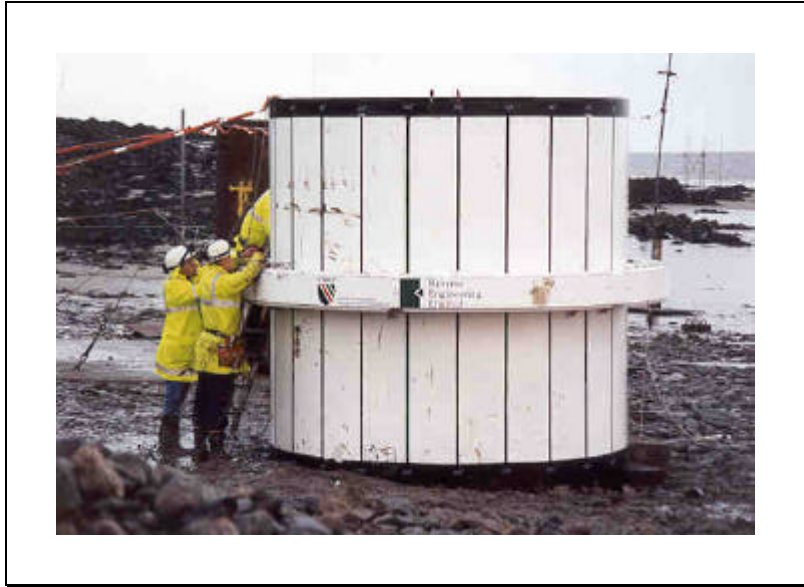
Photo 29. Charge and Tubular awaiting incoming tide
