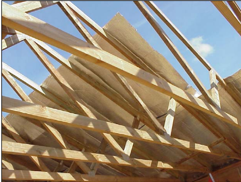
Installation of Radiant Barrier on the Model House.
