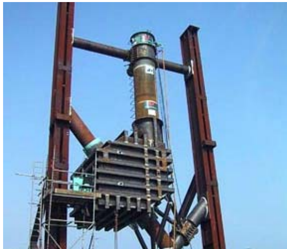
Figure 7.6: Trial fit-up of cofferdam
