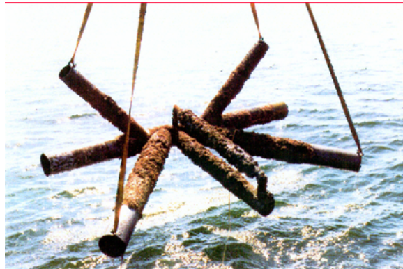
Figure 8.4: Removal of the damaged joint
