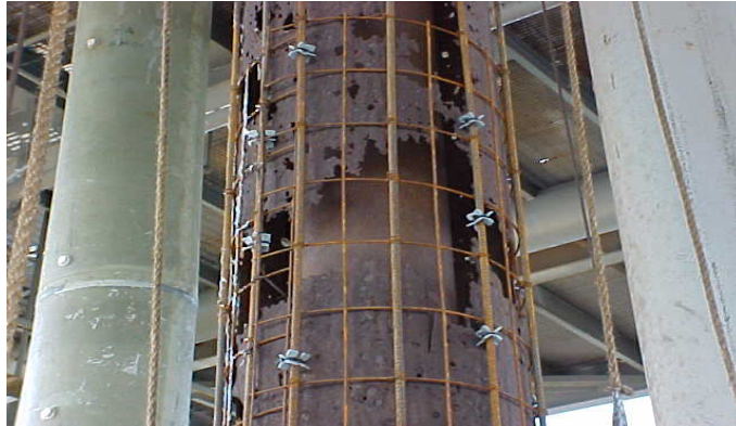
Figure 15.4: Photo of re-bar cage
