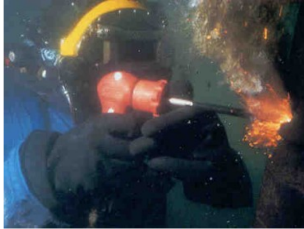
Figure 8.1: Examples of wet welding
