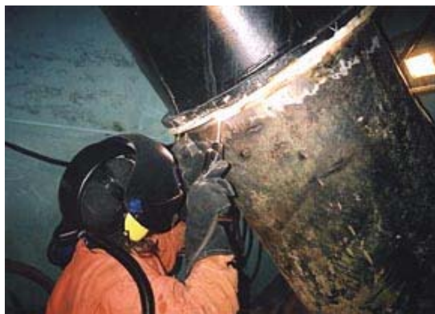
Figure 7.8: Welder at work in cofferdam
