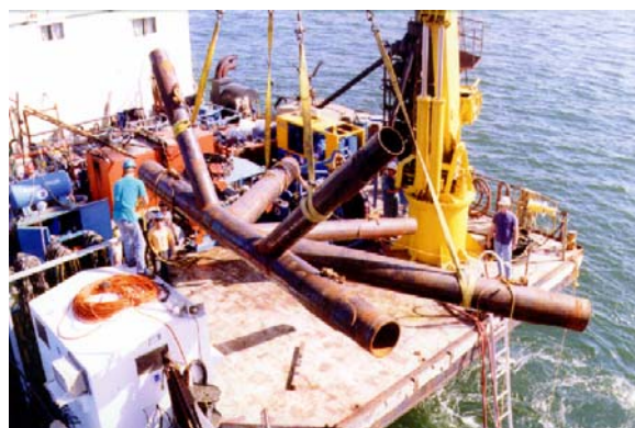
Figure 8.5: Installation of new joint
