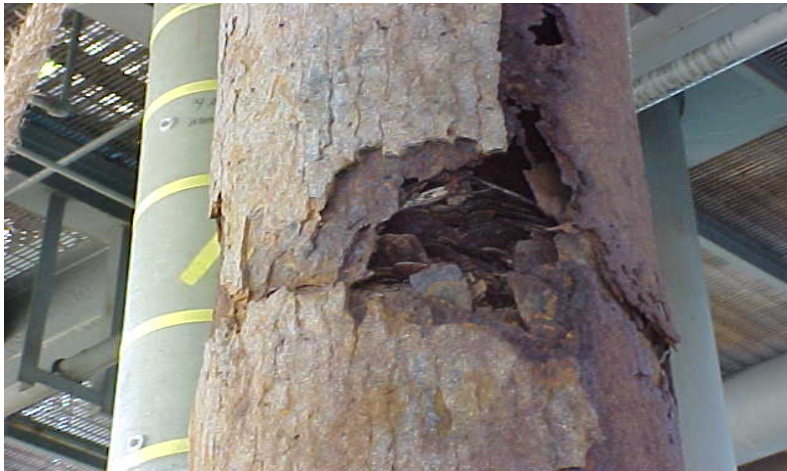
Figure 15.2: Photo of heavily corroded conductor
