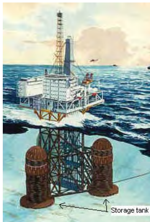
Figure 2.3. Maureen GBS with Three Oil Storage Tanks (Phillips 66 2002)
