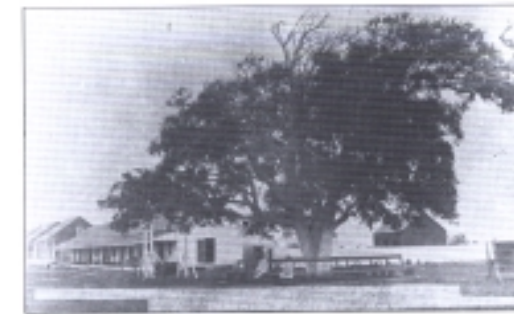
The Kranz Hotel was Grand Isle's first major hotel and was described as an "old, popular, well known resort, built like a plantation quarters, in a series of [38] cottages along a grassy street" (Cole, 1892a, p. 12), no date; (Historic New Orleans Collection, Museum/Research Center, Accession No. 1981.251.11).
