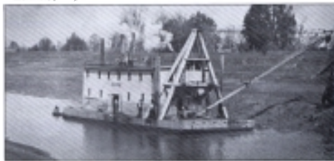
To maintain navigability many bays were dredged, or canals were cut to connect existing waterways. The dredge Eclipse was active in Lafourche and Terrebonne parishes, no date: (Historic Lafourche Collection, Allen Ellender Memorial Library Archives, Nicholls State University, Thibodaux, Louisiana).
