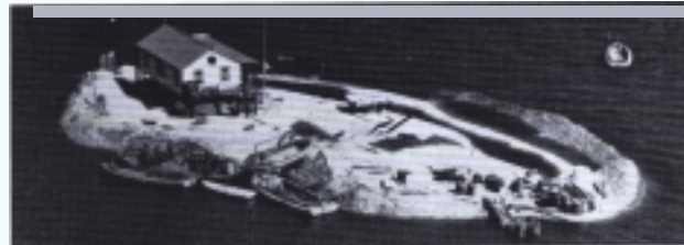
Oystermen often built homes on bird-like wooden legs, two meters above the water; oyster shells thrown around the camp created an artificial island, 1940; Justin F. Bordenave, ed., Jefferson Parish Yearly Review, Special Collections Division, Hill Memorial Library, Louisiana State University Libraries, p. 72.
