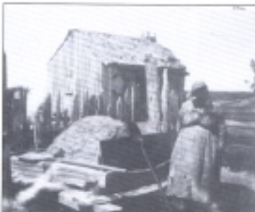
Fisherman's wife next to a typical south Louisiana outdoor (bousillage) oven, which could hold up to 15 loaves of bread at a time, 1891: (National Archives, Negative No. 22-FCD-37).
