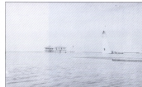
The "floating" Chandeleur lighthouse after the 1893 storm leveled the island, ca. 1893: (National Archives, Negative No. 26-LG-35-47A).
