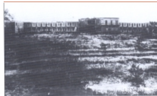
The 1893 hurricane severely damaged The Ocean Club. Built for an estimated $100,000, the facility was never rebuilt in its original grand manner, ca. 1893; (in Mark Forrest, Wasted by Wind and Water: a Historical and Pictorial Sketch of the Gulf Disaster , Milwaukee, Art Gravure and Etching Company, Louisiana Lower Mississippi Valley Collections, Hill Memorial Library, Louisiana State University Libraries).
