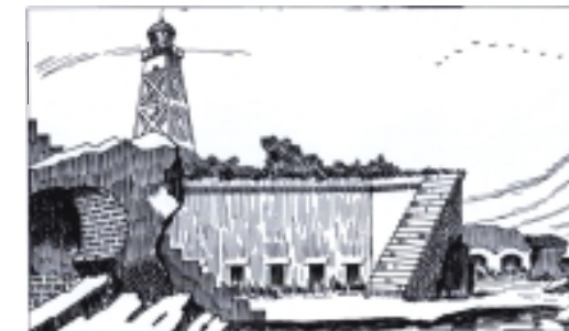
To build Fort Livingston, brick was shipped to the site from the Mississippi Gulf coast. Shells removed from Indian middens were also utilized. With time and the elements the structure became a derelict relic of the past, ca. 1933: (Pen and ink postcard drawing by George Izvolsky).
