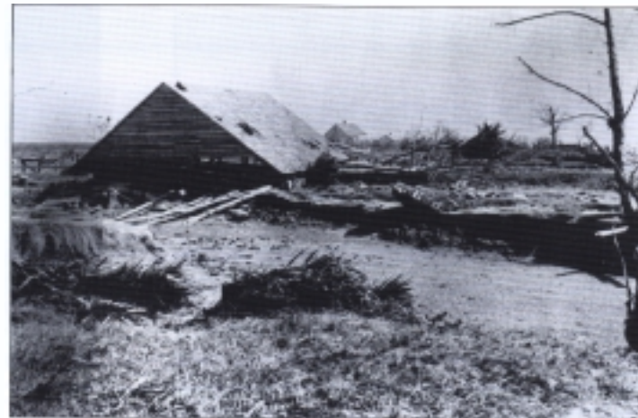
Sixty-two people survived the Cheniere Caminada disaster under the roof of this collapsed shed, no date: (in Mark Forrest, Wasted by Wind and Water: a Historical and Pictorial Sketch of the Gulf Disaster , Milwaukee, Art Gravure and Etching Company, Louisiana and Lower Mississippi Valley Collections, Hill Memorial Library, Louisiana State University Libraries).
