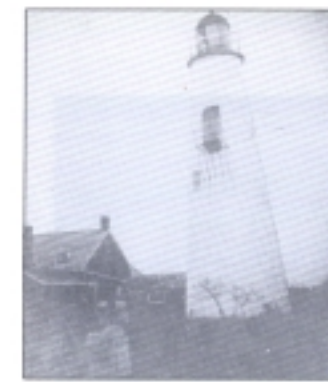
The substantial lighthouse that served traffic navigating Southwest Pass, 1890: (National Archives, Negative No. 26-LG-39-34).
