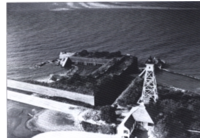
By the mid-1930's the western end of Grand Terre was eroded to the point where the surf was pounding on Fort Livingston's outside walls, date: (Fonville Winans, Louisiana State Library, Louisiana Photographic Archives).
