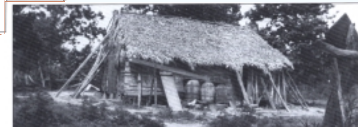
Louisiana's trapper-farmer-fisher folk built their homes from indigenous materials to create functional structures; these were covered with polesetto and equipped with barrel cisterns, ca. 1910; (Sexton Collection, Smithsonian Institution, Photo No. 1536).
