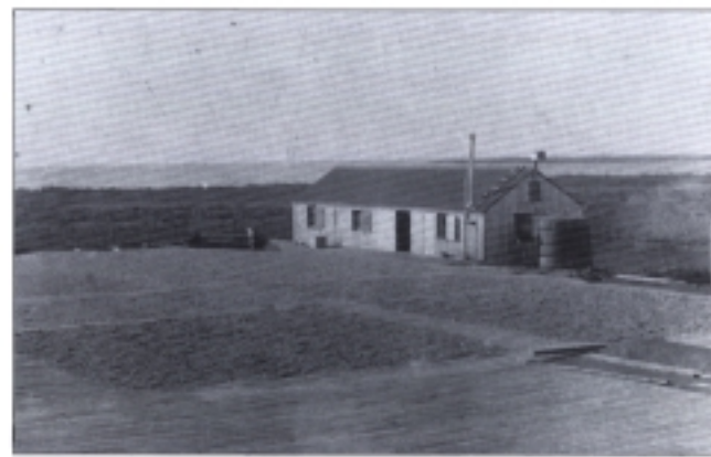
Most shrimp-drying platforms were constructed with cypress. The size of the drying surface varied with each site, but most had a capacity of 1,000 baskets of shrimp—about 50,000 kg, ca. 1920: (Randolph Bazet Collection, Houma, Louisiana)
