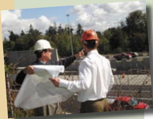
Pete oversees new transportation construction in South King County.
