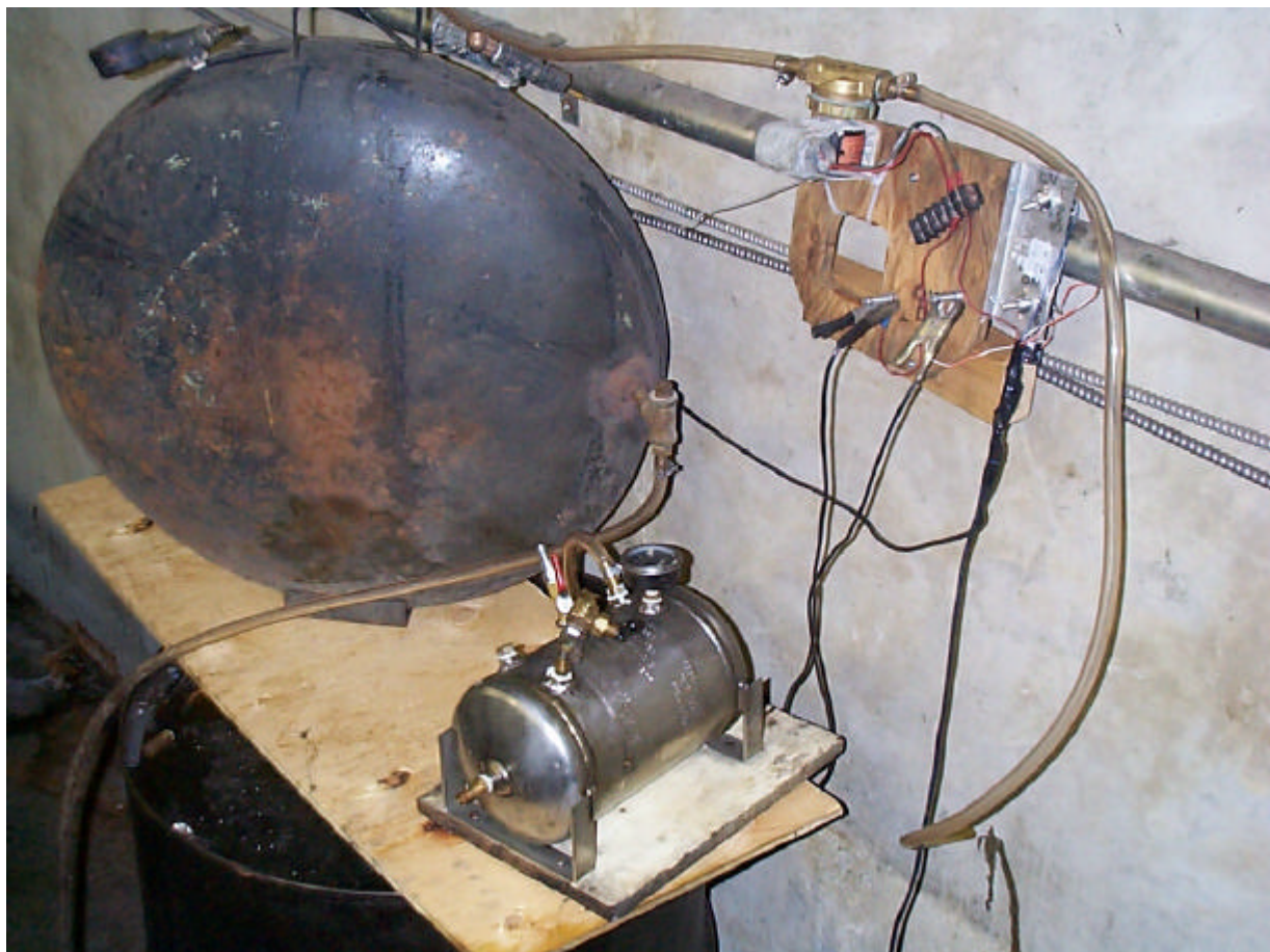
Figure 4: Dispersant Spray Pressure Tanks & Valve
