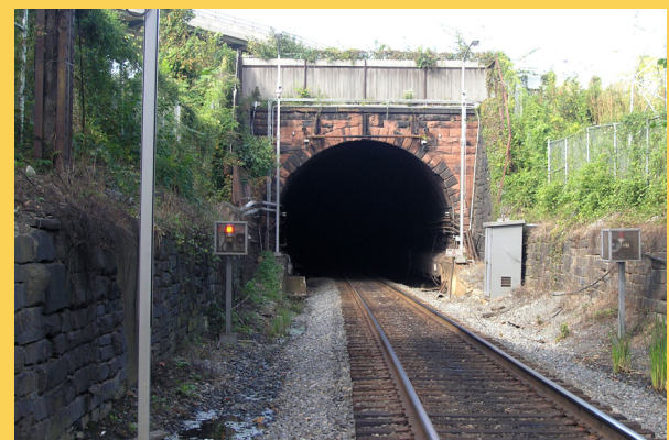
Figure 2-5. Virginia Avenue Tunnel
