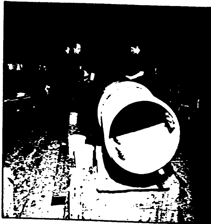
Fig. 10. Cladding of a steel riser with FRP (Courtesy of Vosper Thornycroft (UK) Ltd).
