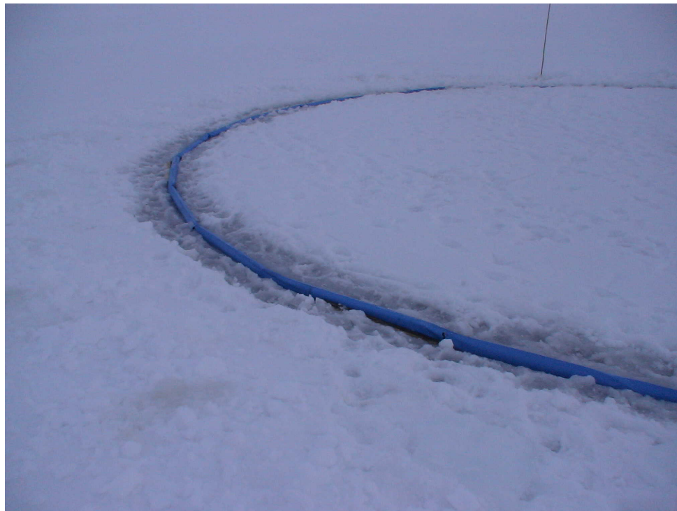
Completed skirt installation
